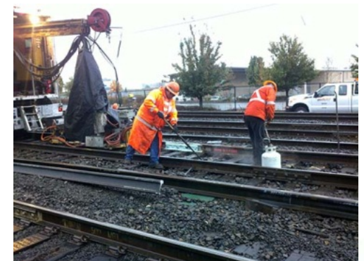
BNSF crews replace worn track near Vancouver, WA
