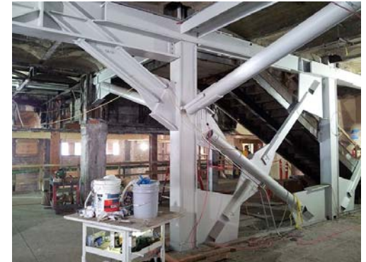
New steel in King Street Station's upper floor
