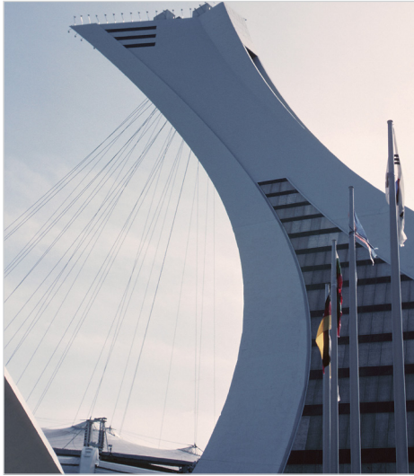
Olympic Stadium Montreal, Canada
