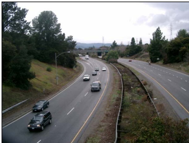
SR 237 looking west towards SR 85
