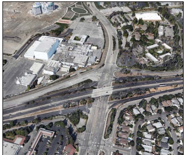
Aerial View of Mathilda Avenue at SR 237
