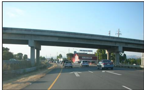
Northbound US 101 at SR 25 Overcrossing
