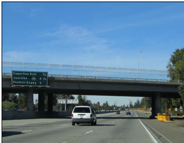
I-280 Northbound, approaching Foothill Expressway
