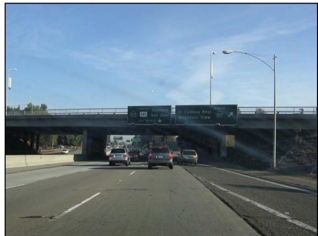
SR 85 Northbound, approaching SR 237/US 101
