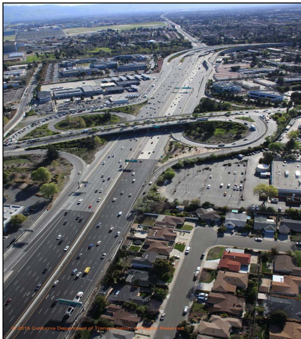
US 101 - Looking south at Shoreline Blvd Interchange
