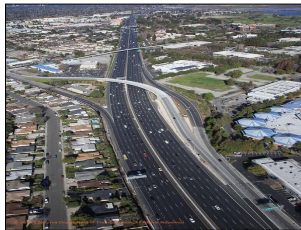
US 101 - Looking north at Old Middlefield Way on and off ramp
