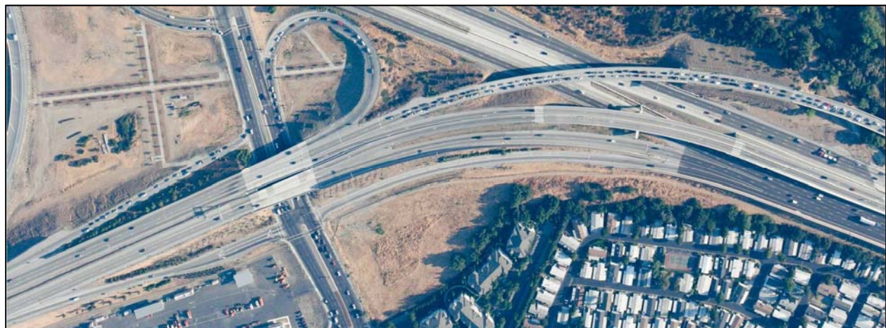
Aerial view of SR 85 - US 101 Interchange in South San Jose
