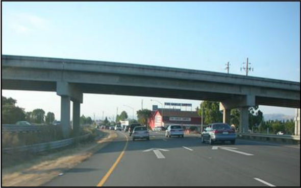
Northbound US 101 at SR 25 Overcrossing
