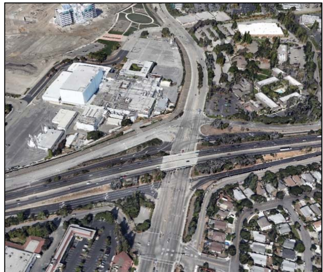
Aerial View of Mathilda Avenue at SR 237
