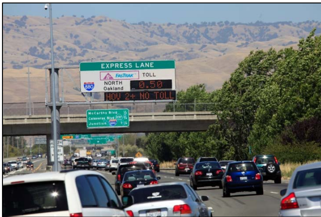
Express Lanes entrance from Eastbound SR 237 Express Lanes
