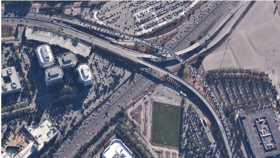
Figure 2-16. Evening Congestion Near Mineta San Jose International Airport (SR 87/US 101/Charcot Avenue)
