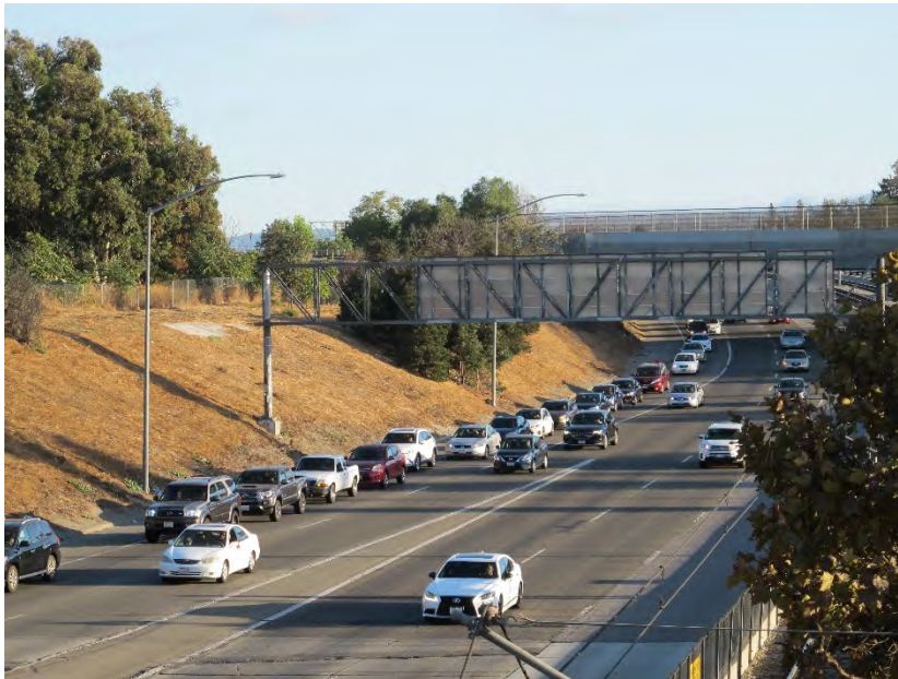
Figure 2-17. Right-Lane Overload on Northbound SR 87 Approaching the I-280 Ramp
