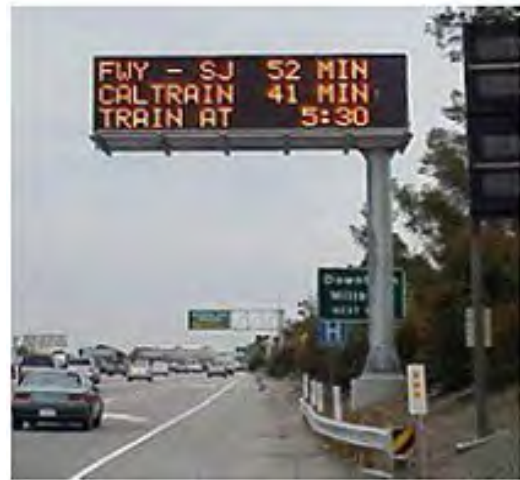
Figure 5-12. Changeable Message Sign Display with Train Schedule and Travel Time Source: ScienceDaily
