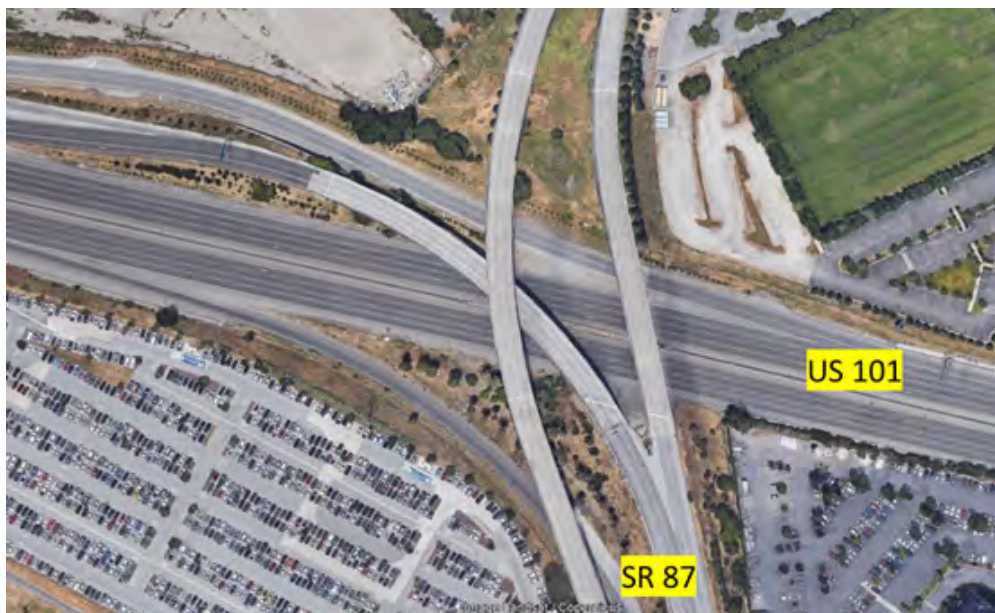
Figure 2-6. SR 87/US 101 System Interchange
