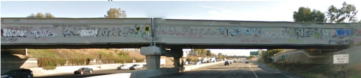
US 101 SB Railroad Trestle Bridge /Old Oakland Rd.
