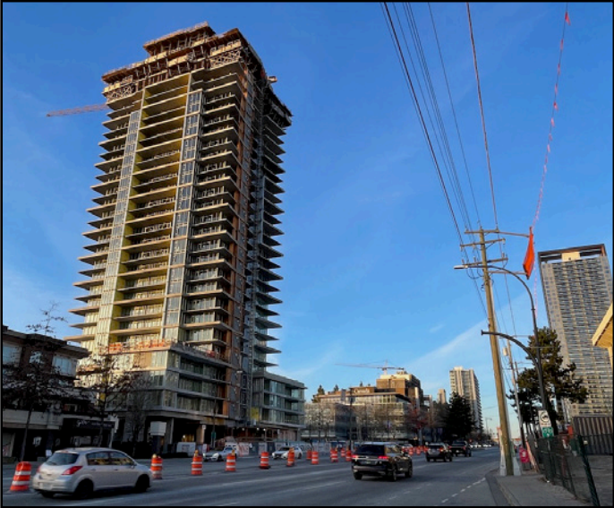
Belvedere - Topped out at final height above King George Blvd
