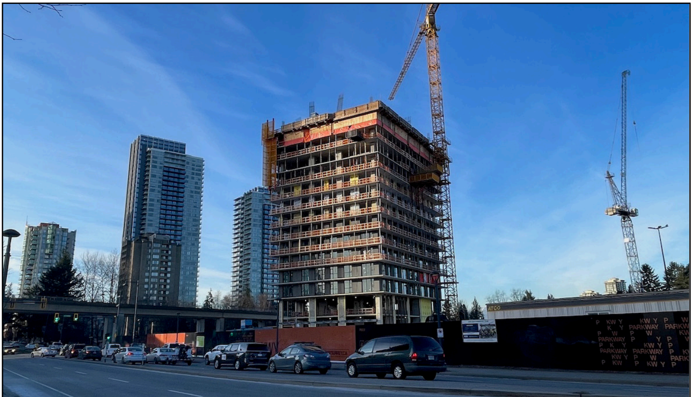
Parkway - Phase 1 rental tower continuing to rise above 104 Ave & City Parkway
