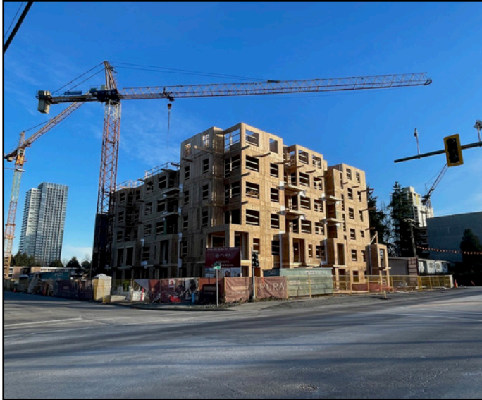
Pura - Beginning to take shape at corner of 105 Ave & 132 St
