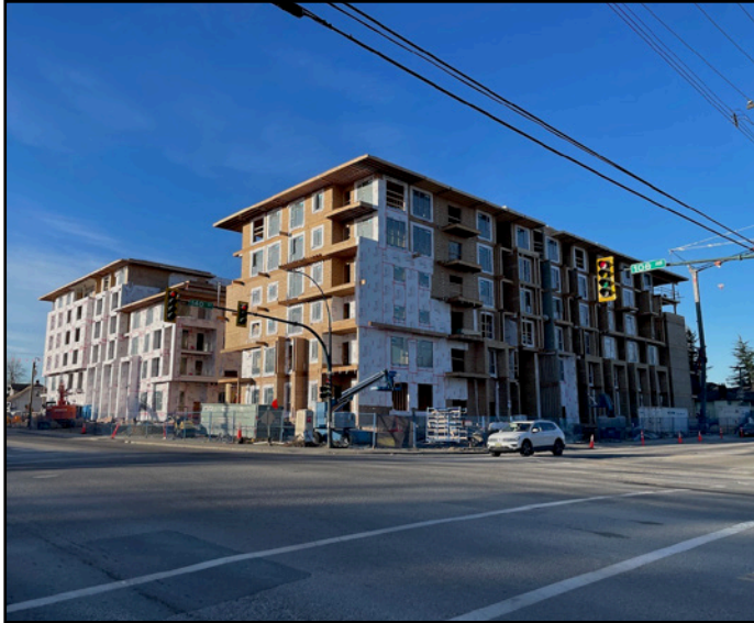
Viktor - Exterior work continues at 108 Ave & 140 St
