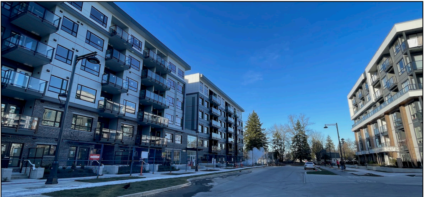
Q5 - Completed in January 2024 at corner of 108 Ave & 138 St
