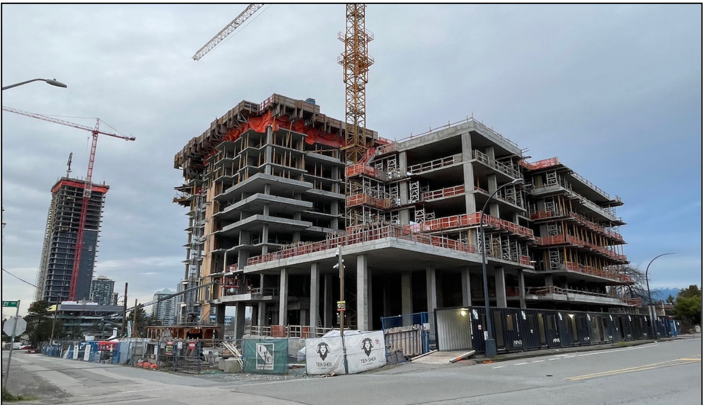
Flamingo One - Residential tower beginning to rise above office podium
