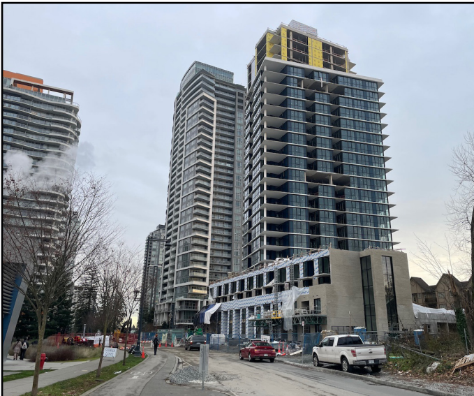
Melrose - Exterior work continuing along Central Ave
