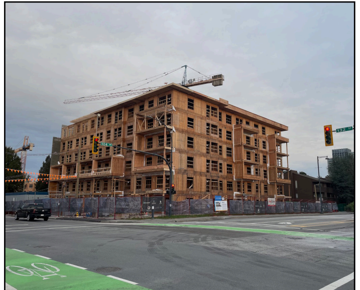
Sunshine Co-op - Continuing to take shape at 104 Ave & 132 St
