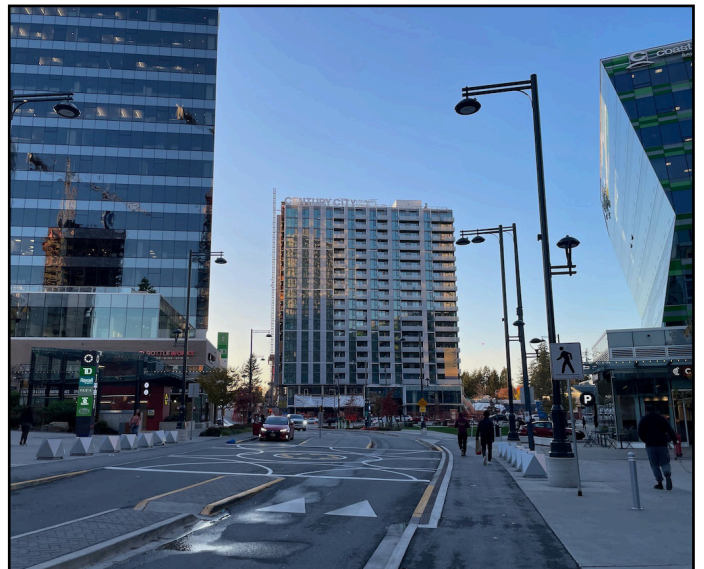
Century City - Exterior work continues on 19-storey rental tower
