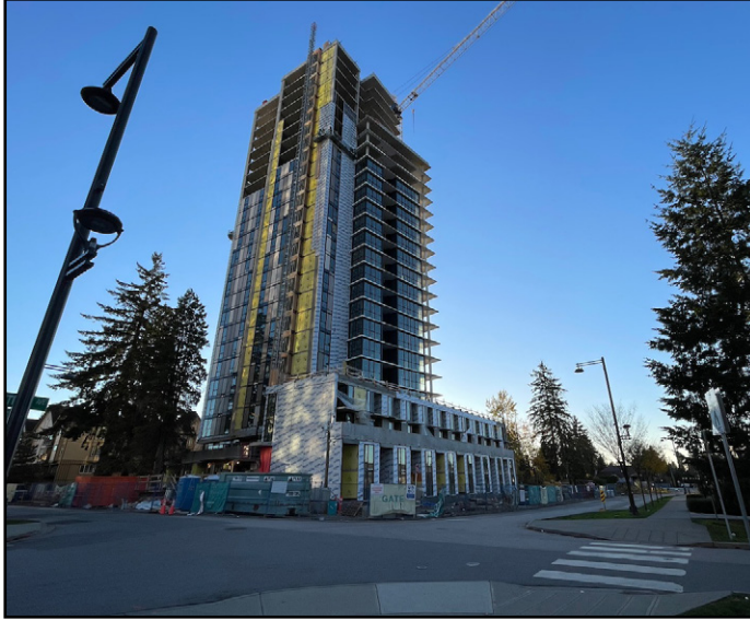
Melrose - Now topped out at 26-Storeys above Central Ave & 133 St
