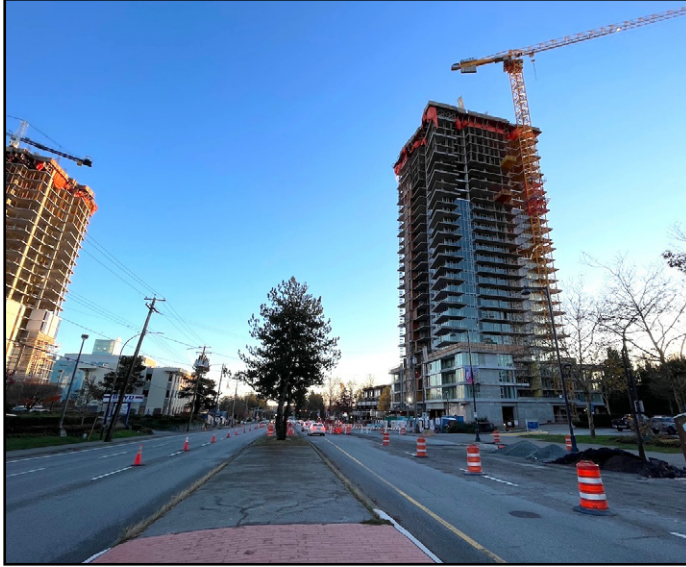
Belvedere - Nearing final height of 27-storeys along King George Blvd
