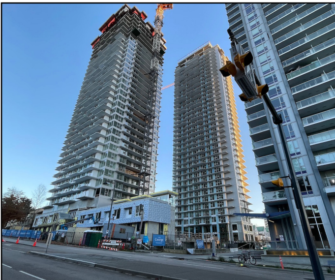
Park George - Towers now topped out at 35 & 39-Storeys along 100 Ave
