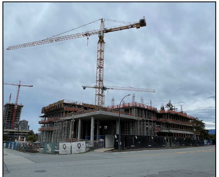
Flamingo One - Tower beginning to rise behind office podium
