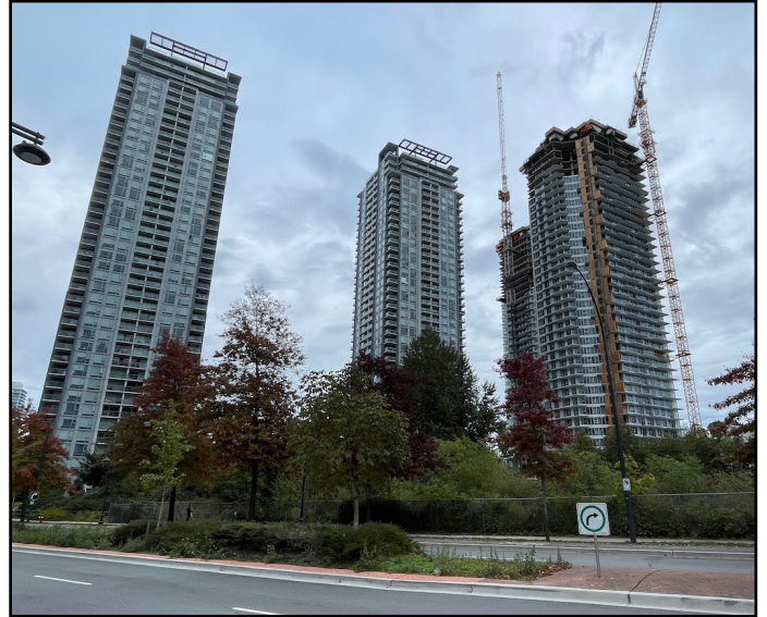
Park George - Both towers now topped out at 35 & 39-Storeys
