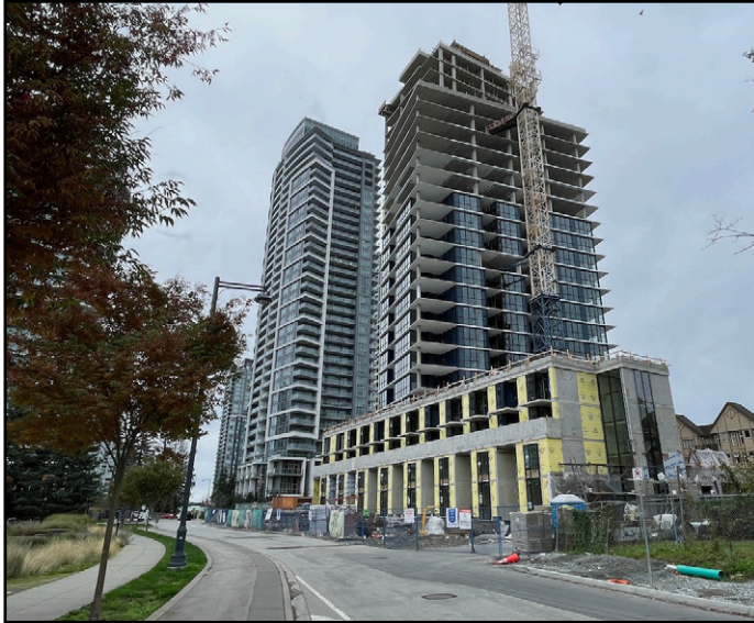
Melrose - Tower now topped out at 26-storeys
