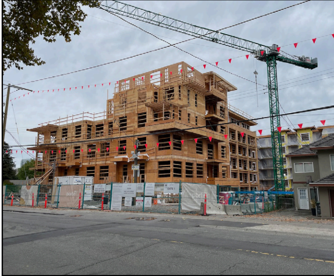
Quinn - Framing taking shape along 134 St
