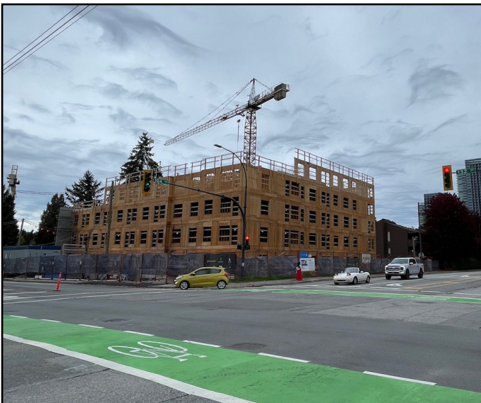
Sunshine Co-op - Framing taking shape at 132 St & 104 Ave
