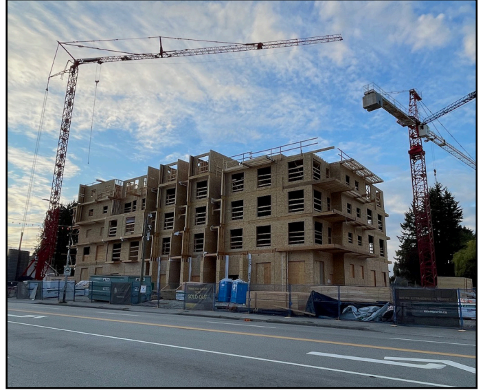
Victor - Framing taking shape along 108 Ave
