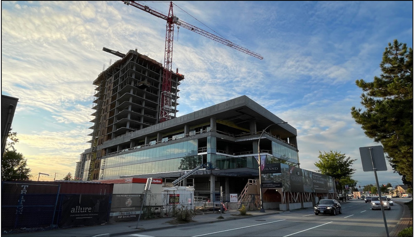
The Grand - Glazing installation underway on office podium
