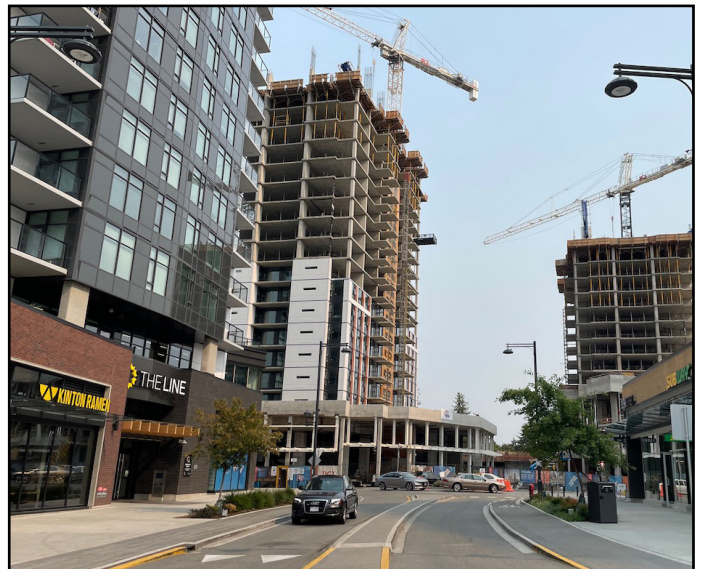
Plaza One & Two - Continuing to rise above George Junction
