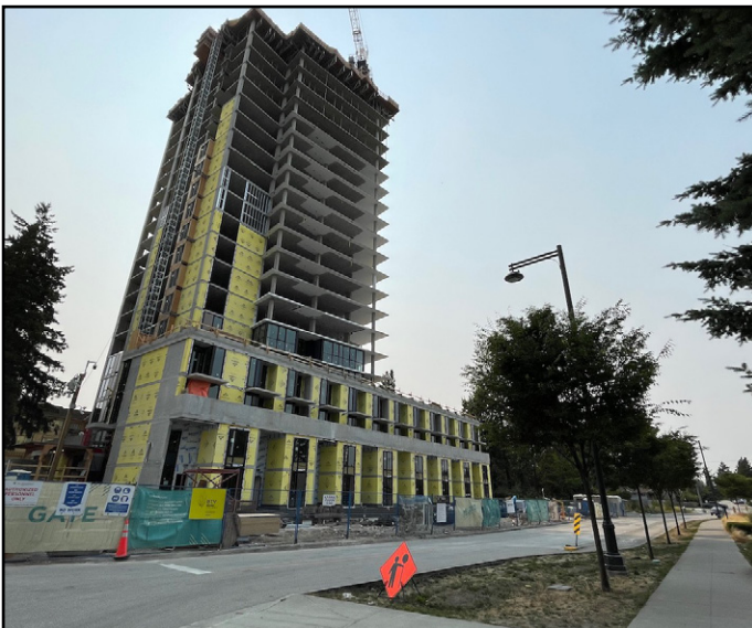
Melrose - Tower continuing to rise above Central Ave
