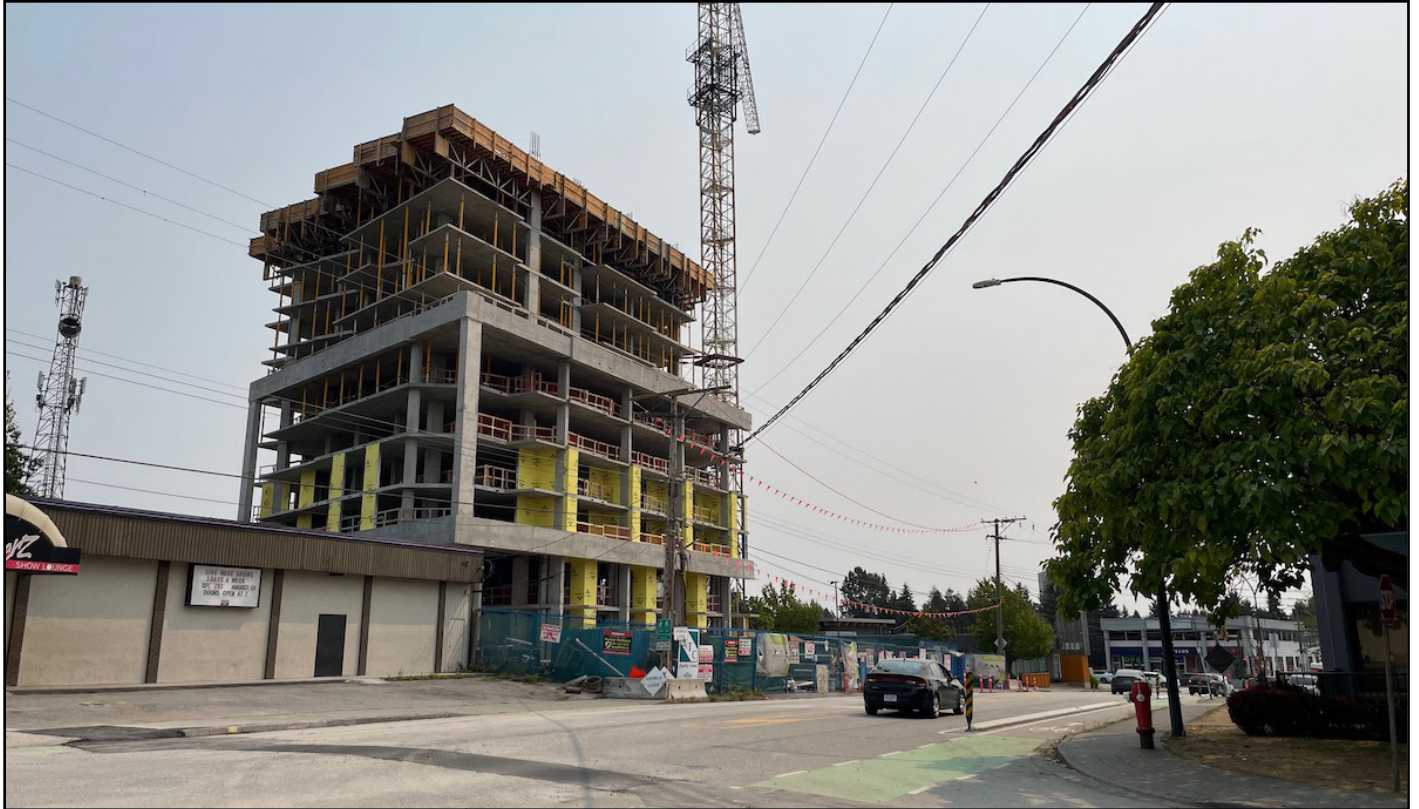
Ascent - Tower beginning to gain height above podium along Whalley Blvd
