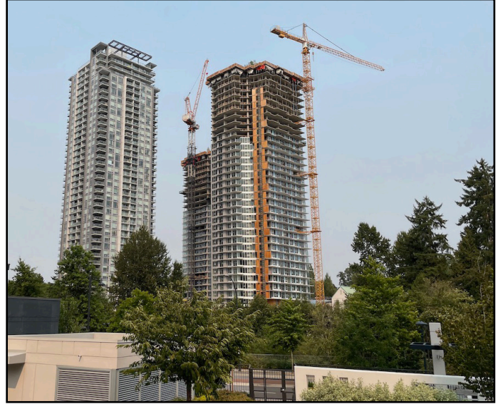
Park George - Towers continuing to gain height
