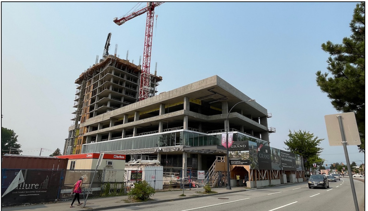
The Grand - Main tower gaining height above office & retail podium
