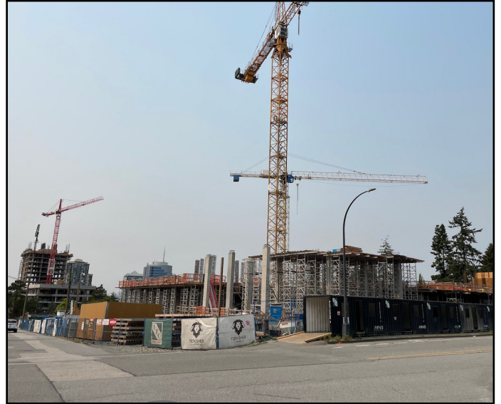
Flamingo One - Podium taking shape along Whalley Blvd
