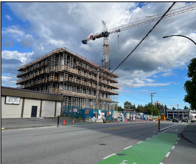
Ascent - Tower beginning to rise above Whalley Blvd
