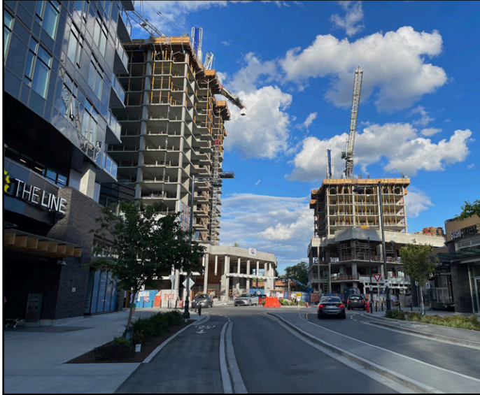
Plaza One & Two - Towers beginning to rise at King George Hub
