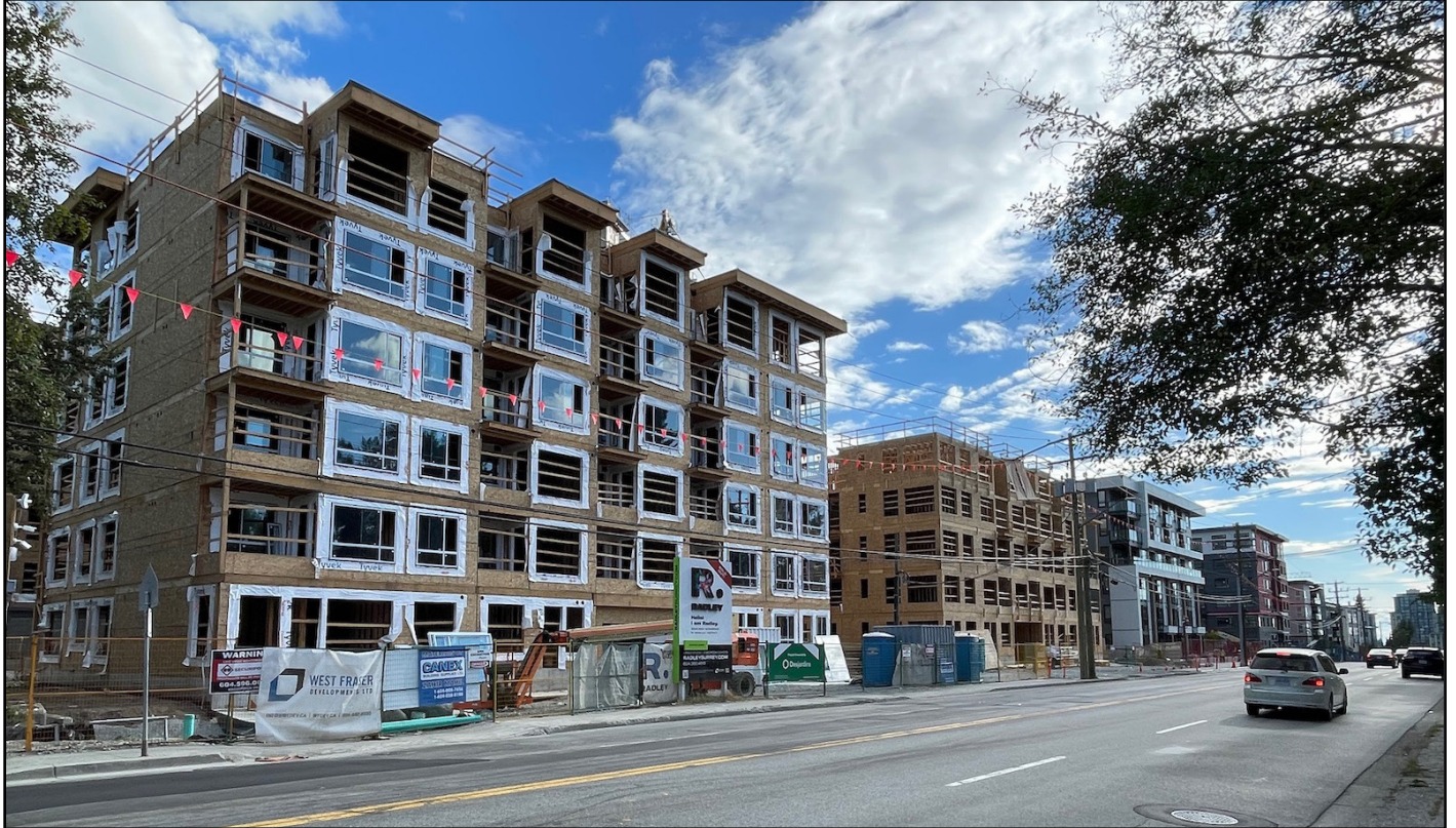
Radley / Hendrix / Q5 - Trio of 6-Storey projects re-shaping the 108 Ave corridor
