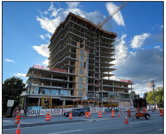
Belvedere - Tower continuing to rise above King George Blvd
