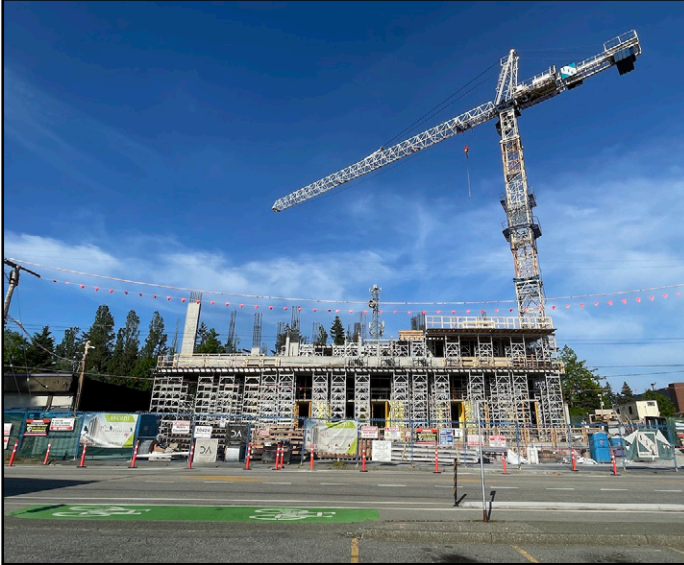
Ascent - Podium levels construction underway along Whalley Blvd
