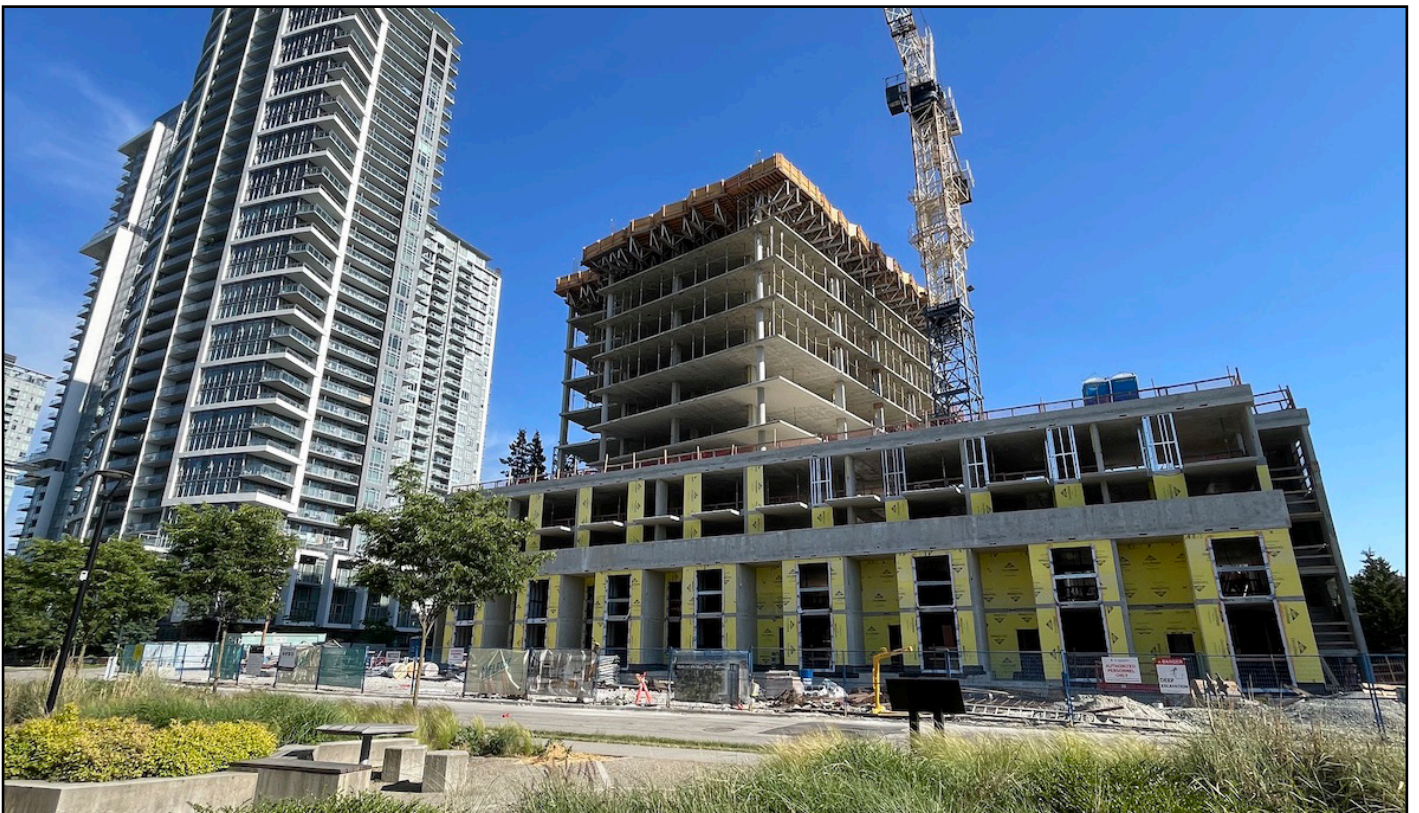
Melrose - Tower beginning to rise above podium along Central Ave
