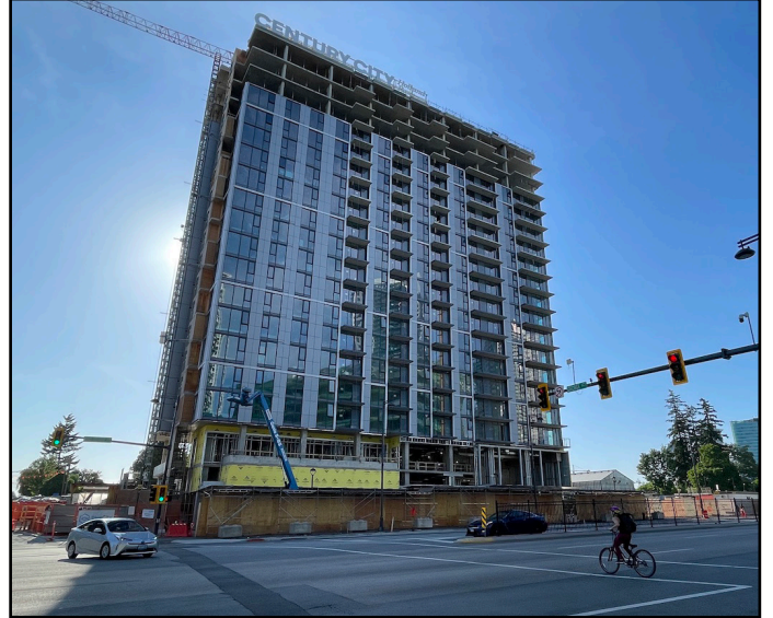
Century City - Rental tower now topped out at King George & 98 Ave
