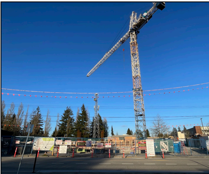
Ascent - Parking levels construction nearing grade
