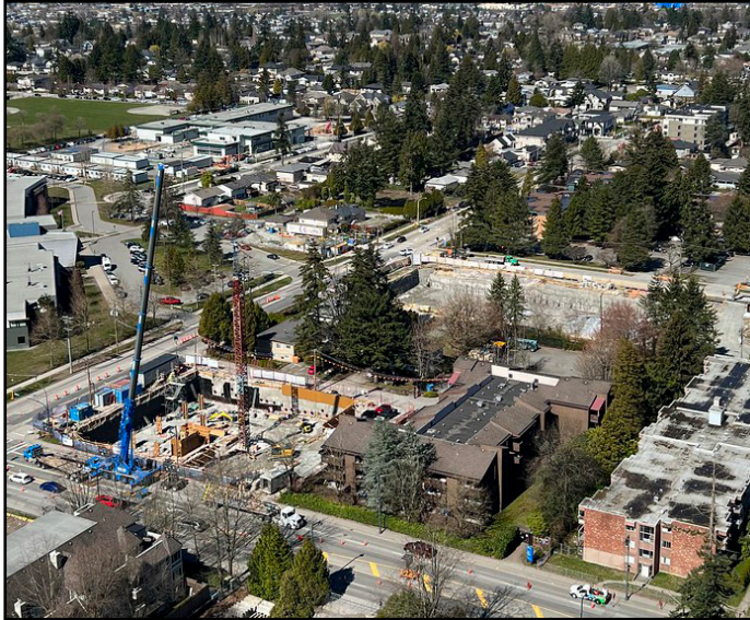
Sunshine Co-op & Pura - Crane installation and excavation underway
