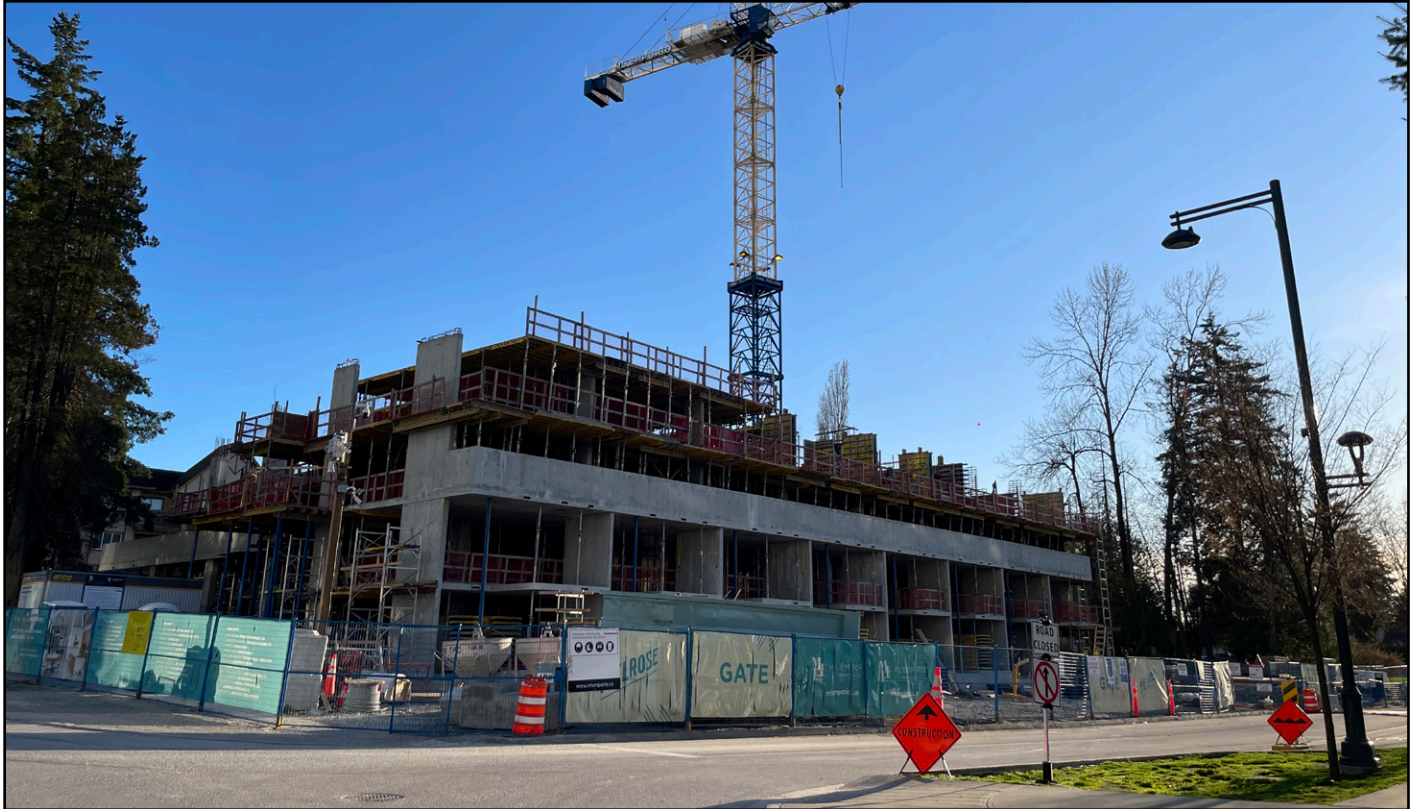
Melrose - Podium levels taking shape with street-oriented townhomes along Central Ave
