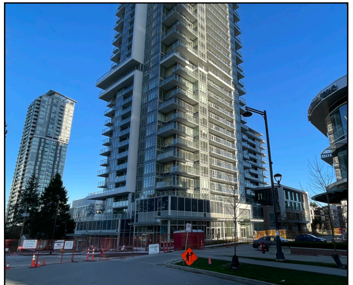
One Central - Nearing completion
