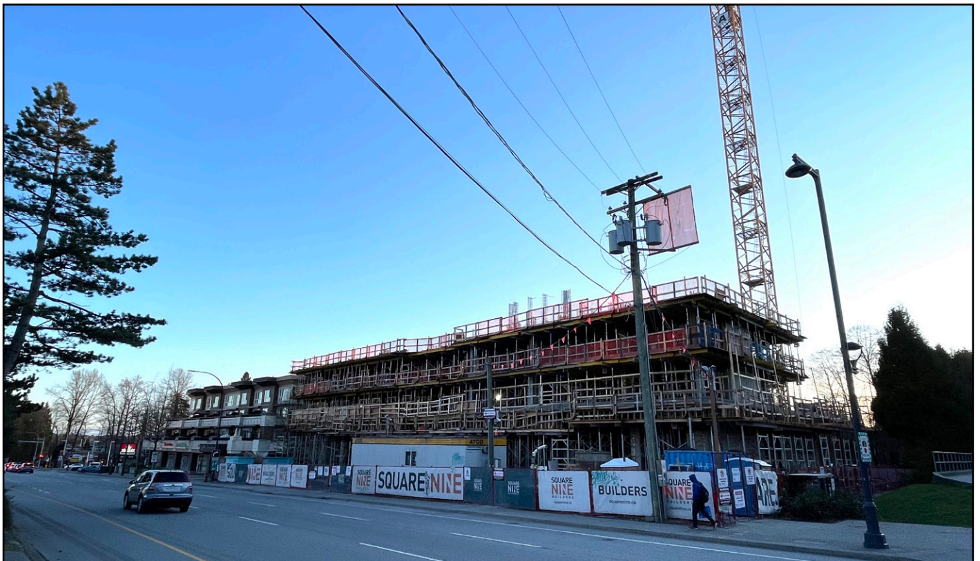
Belvedere - Podium levels taking shape along King George Blvd
