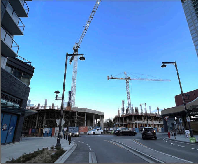
Plaza One & Two - Podium levels continue to rise
