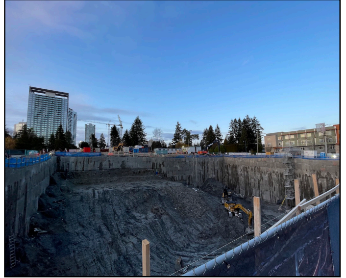
City Centre 4 - Excavation progressing
