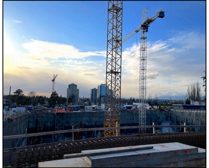
Flamino One - Parking levels construction underway
