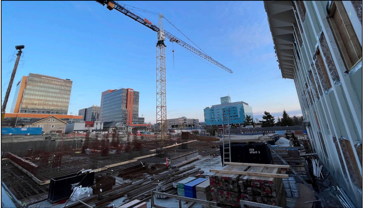
Comma King George - Parking levels construction underway and nearing grade
