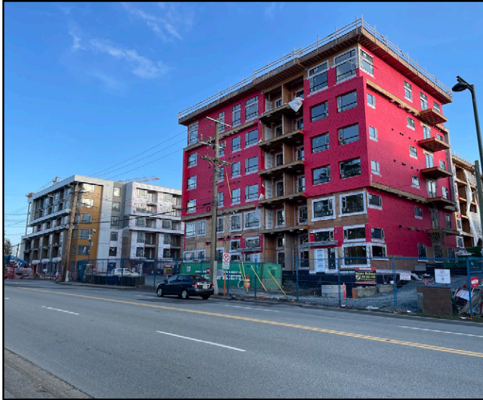
Q5 & Hendrix - Exterior work continues
