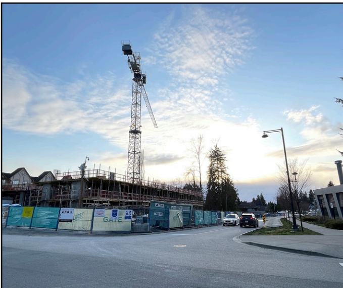
Melrose - Podium levels beginning to rise above grade
