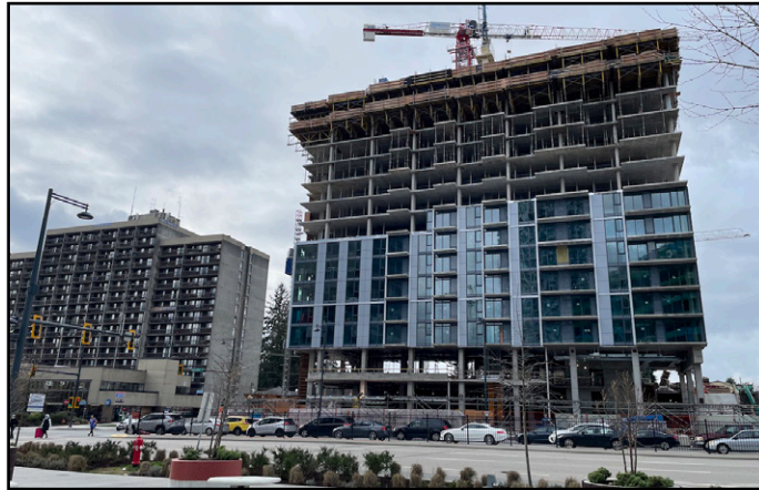
Century City - Rental tower continuing to rise
