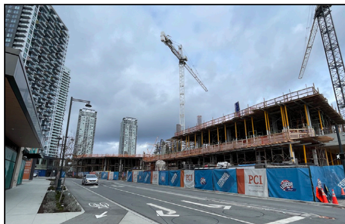
Plaza One & Two - Retail / office podium taking shape
