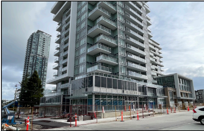
One Central - Nearing completion
