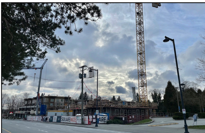
Belvedere - Beginning to rise above grade
