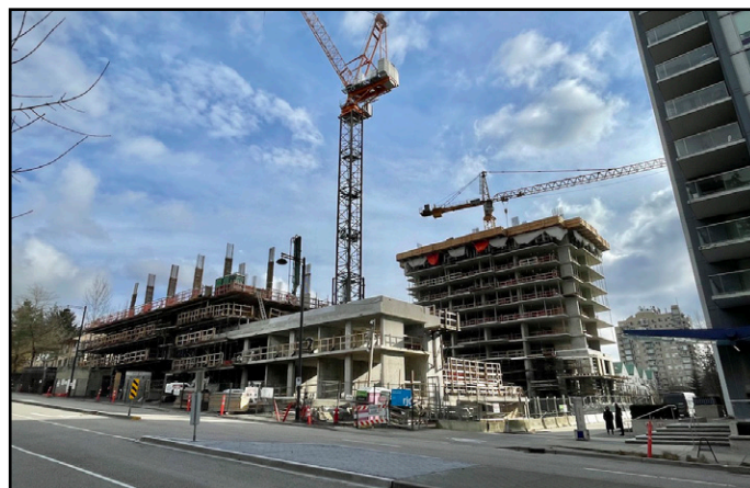
Park George - Towers and podium beginning to take shape
