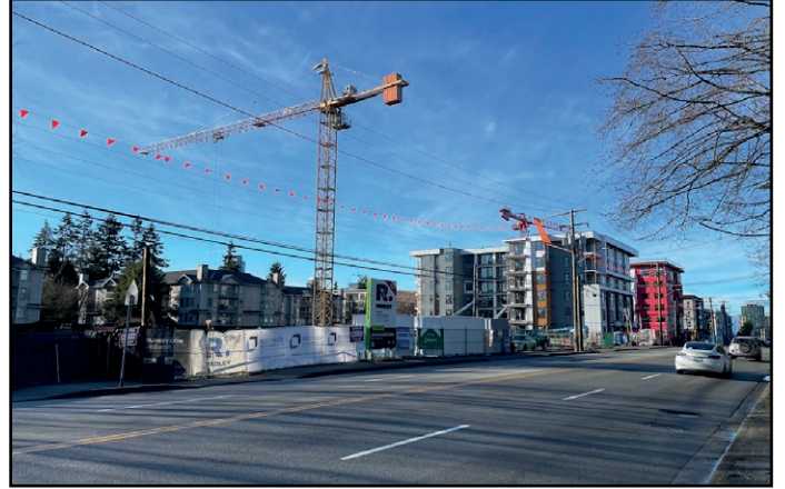
Radley, Hendrix, & Q5 - Crane for Radley now up along 108 Ave
