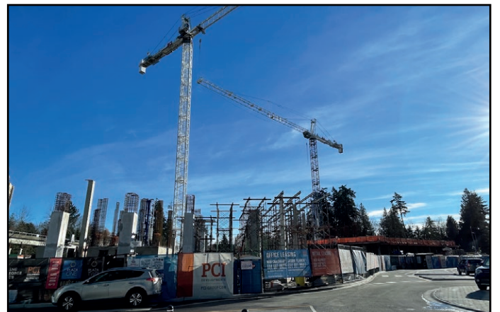
Plaza One & Two - Beginning to rise above grade
