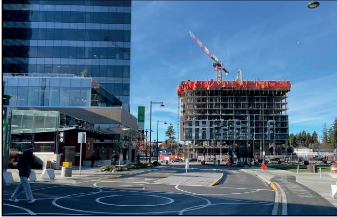
Century City 1 - Glazing installation underway on rental tower
