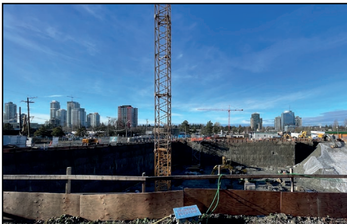
Flamingo One - Crane now installed with work beginning on parking levels
