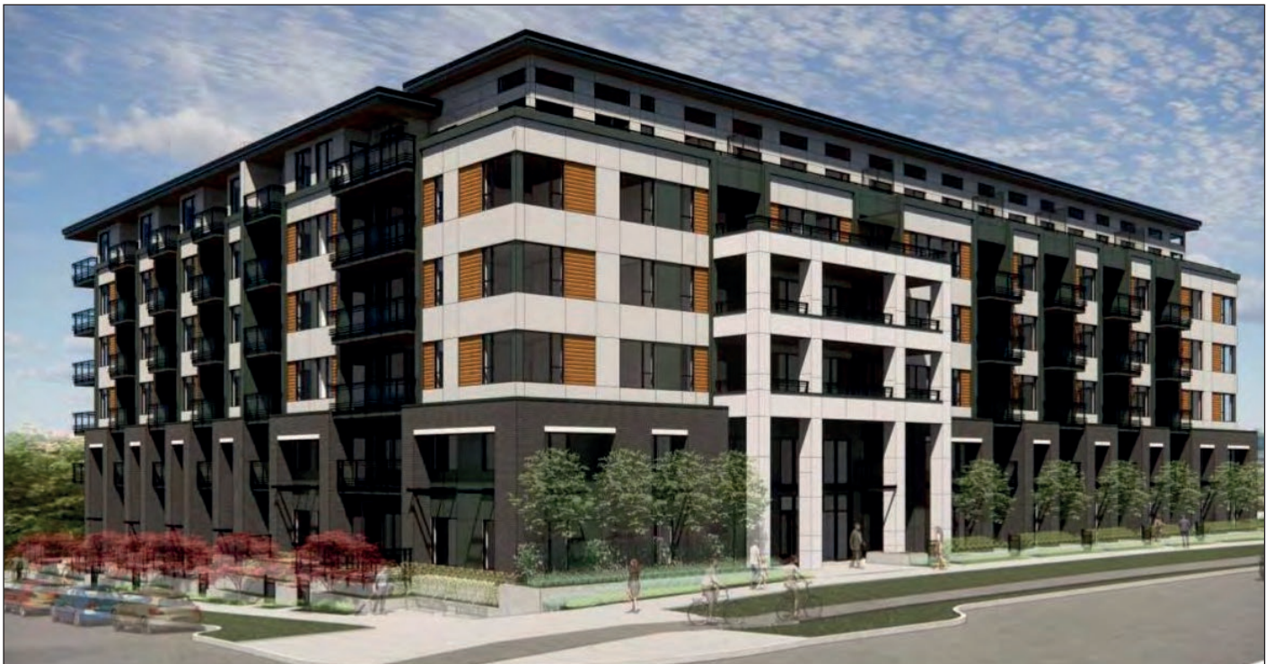
View looking south-east from corner of 134 St & 95 Ave
