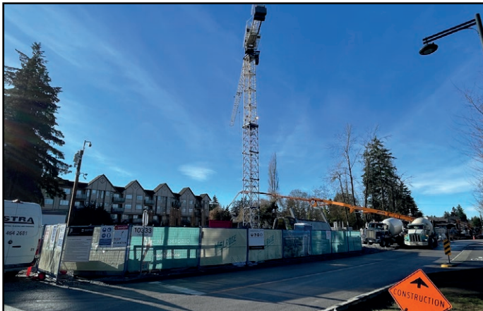
Melrose - Parking levels construction nearing grade
