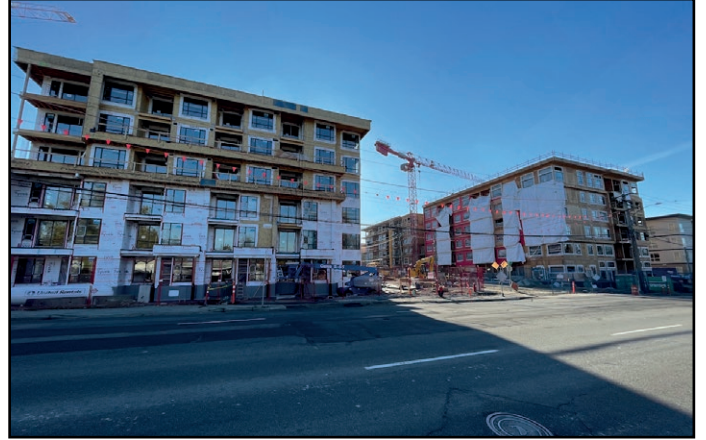
Hendrix & Q5 - Now topped out along 108 Ave
