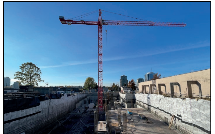
The Grand - Parking levels construction nearing grade
