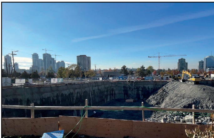
Flamingo One - Excavation progressing
