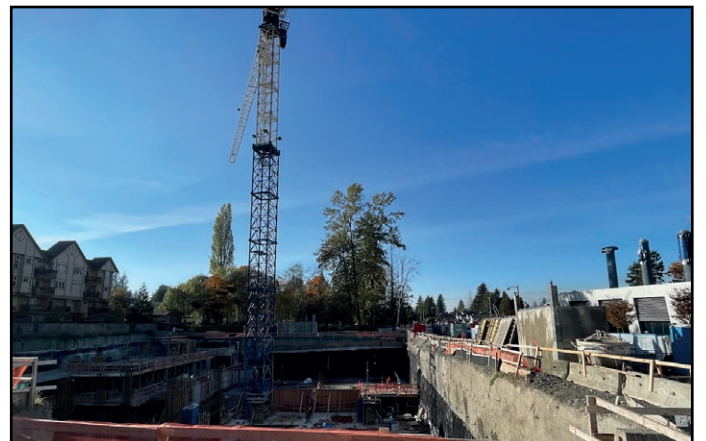
Melrose - Parking levels construction nearing grade
