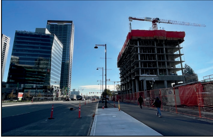
Century City 1 - 19-Storey Rental Tower gaining height
