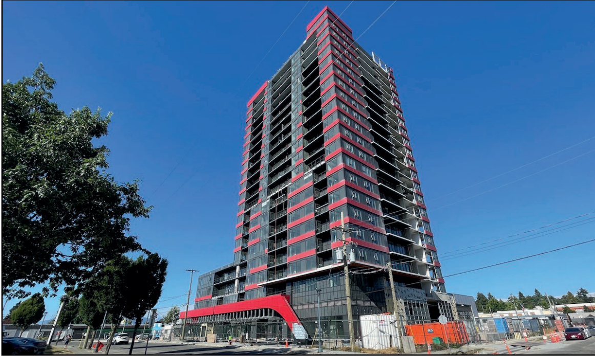
Parc Centrale - Exterior work nearing completion
