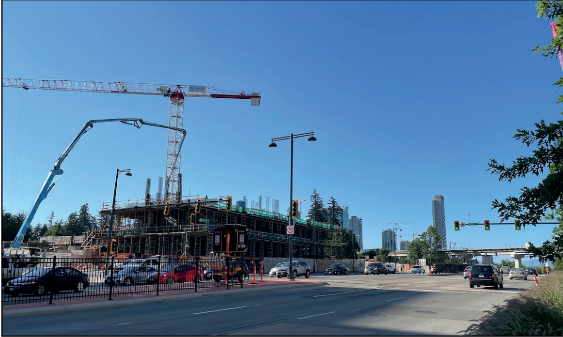
Century City - Work beginning on 3rd level of 19-storey rental tower
