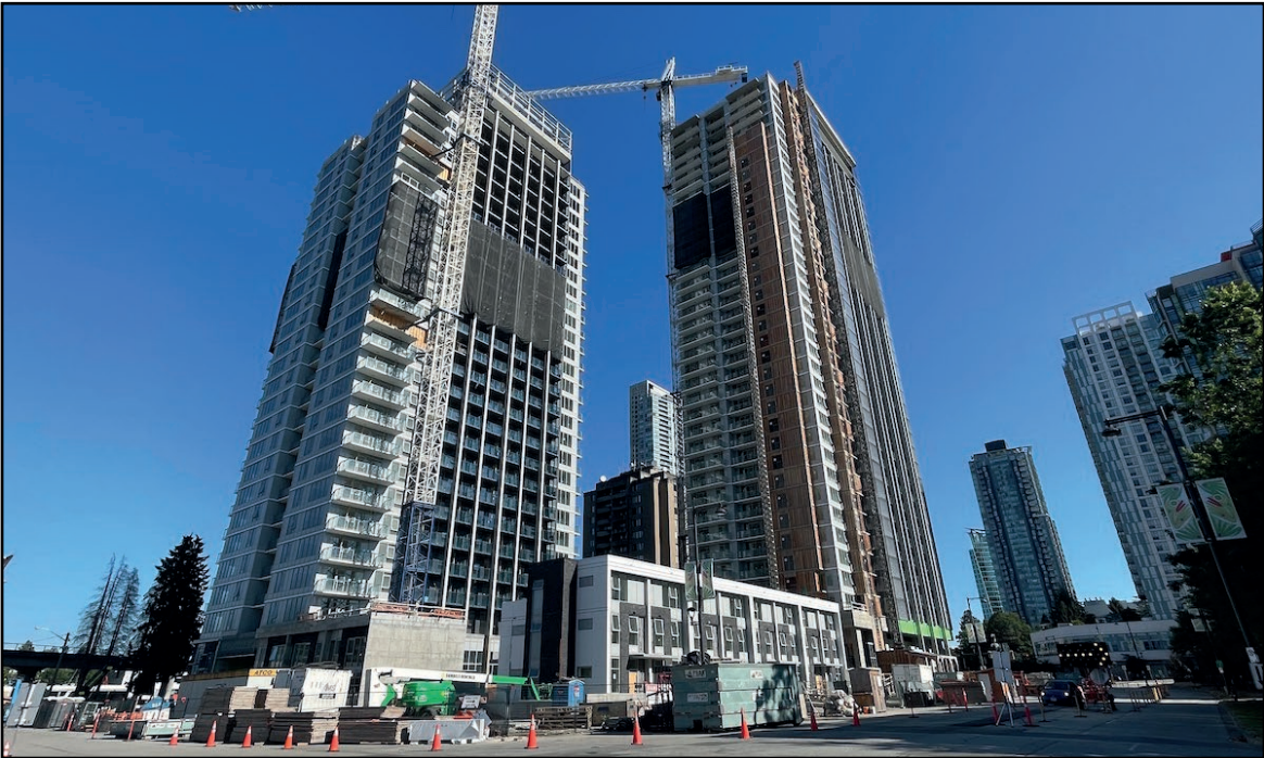
University District - Both towers now topped out at 28 & 37-storays
