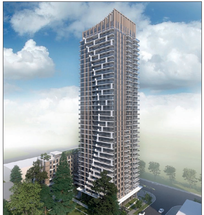
View looking north-west from 133 St
