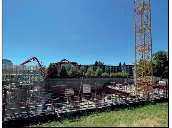
Belvedere - Parking levels construction continues
