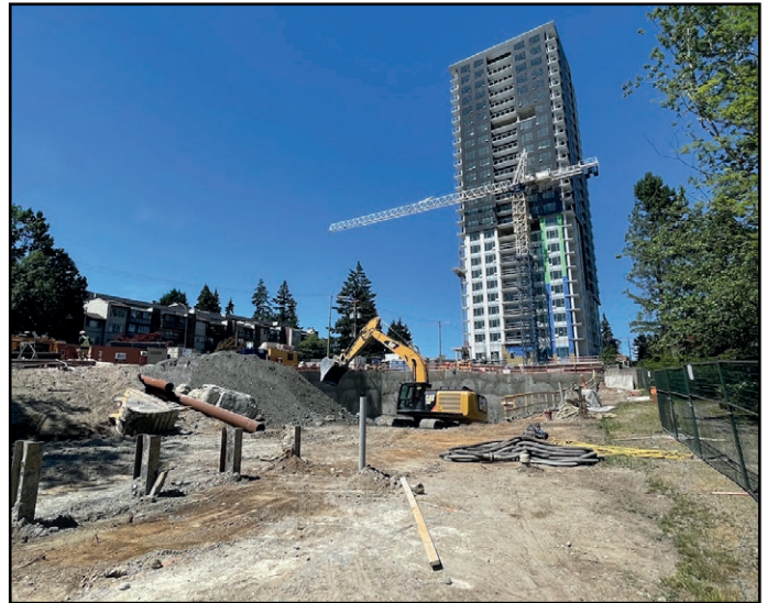
The Holland Two - Excavation underway
