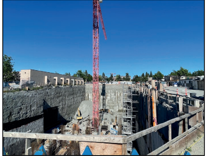
The Grand - Work beginning on parking levels
