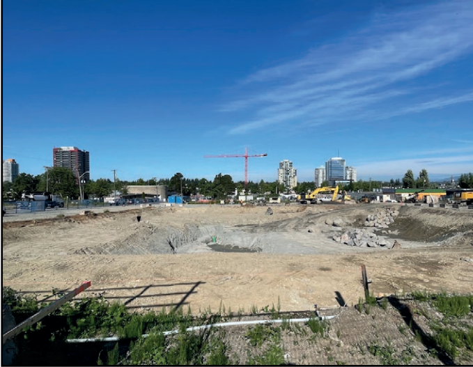
Flamingo One - Early stages of excavation underway
