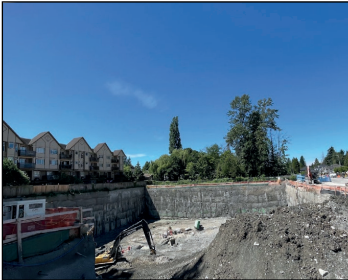
Melrose - Excavation progressing
