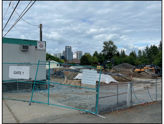
Quinn - Excavation beginning
