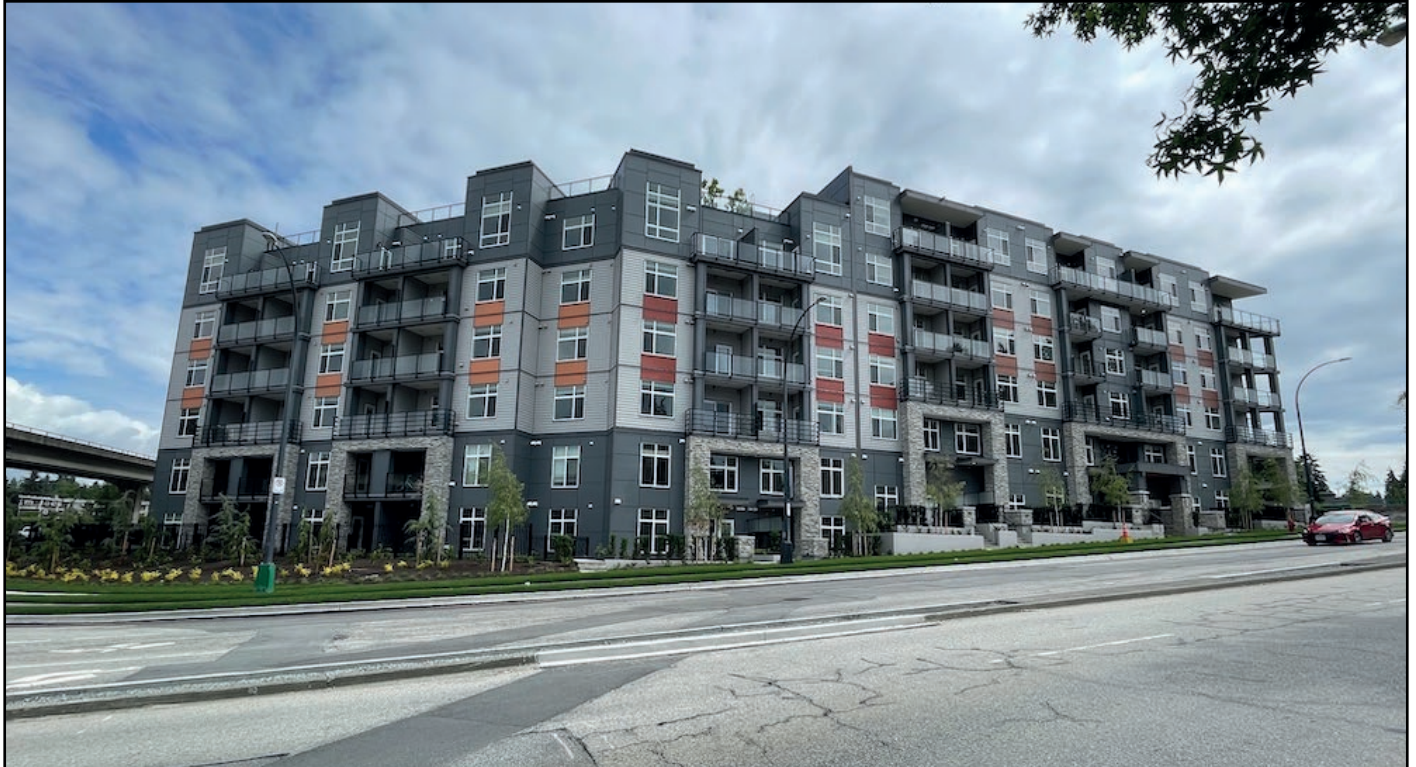
Ledgview - 6-storey condo building now complete at 132 St & King George Blvd
