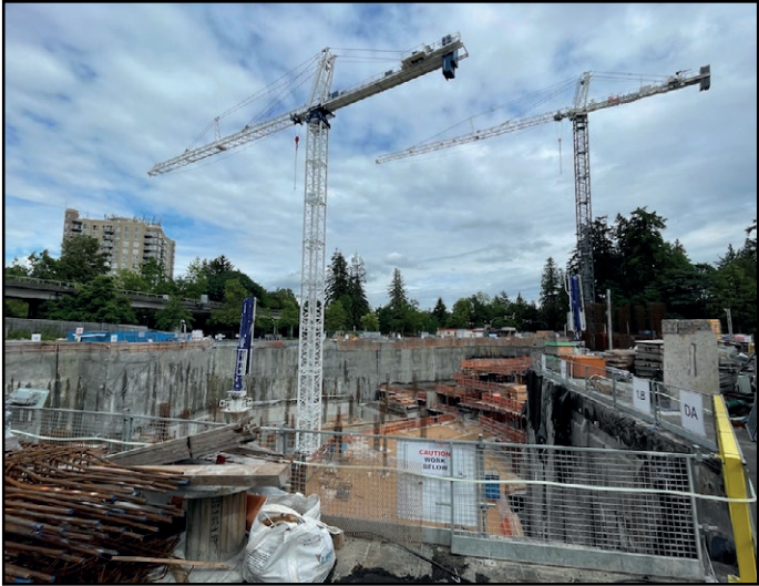
Plaza One & Two - Parking levels construction continues
