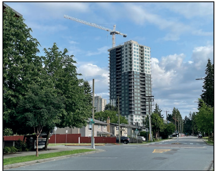
The Holland - Now topped out with exterior mostly complete
