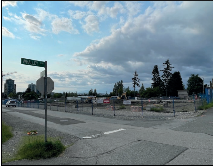
Flamingo One - Site preparation now underway
