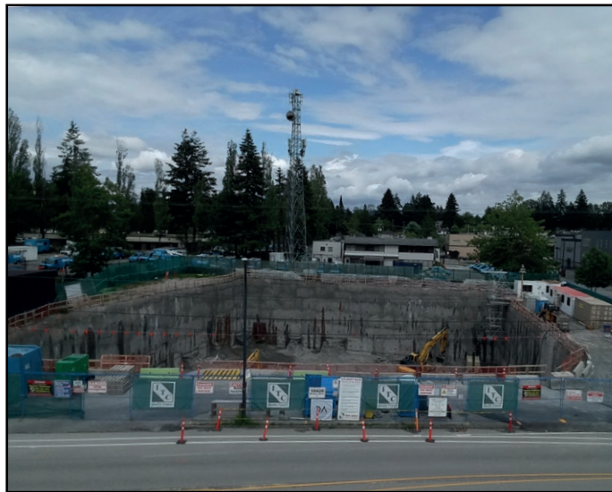
Aspect - Excavation continues
