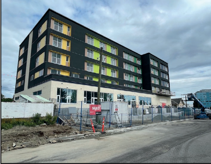
Rosewood - Exterior work nearing completion
