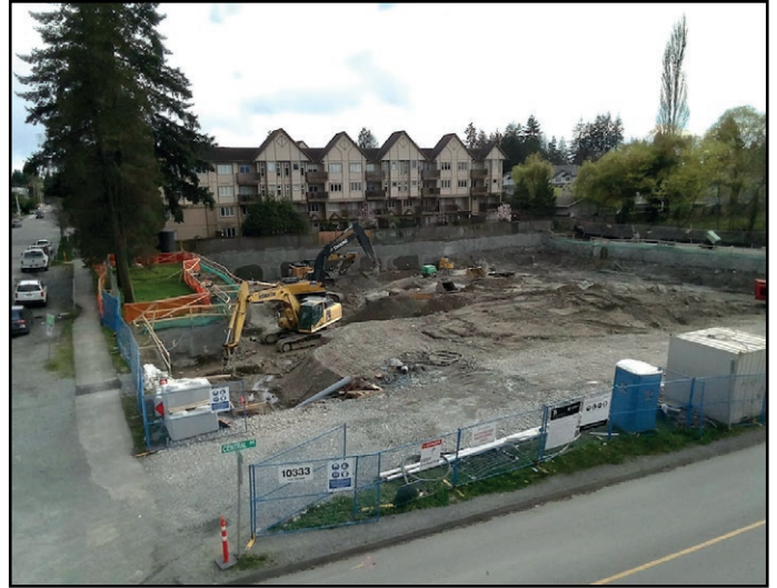
Melrose - Excavation progressing
