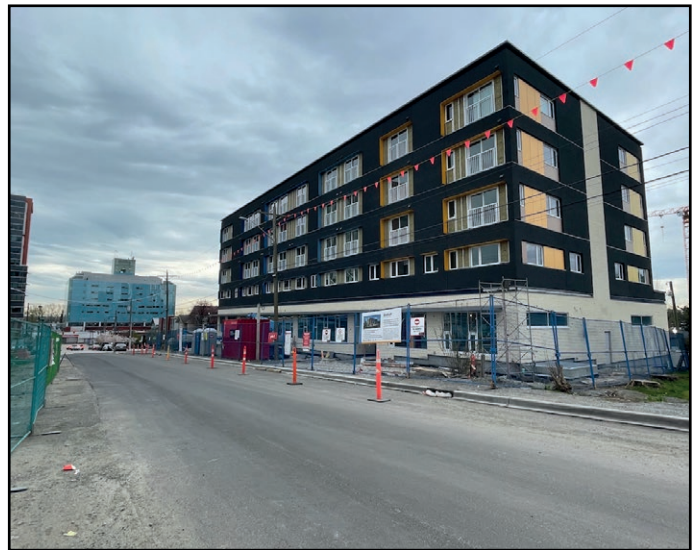
Rosewood - Exterior cladding progressing
