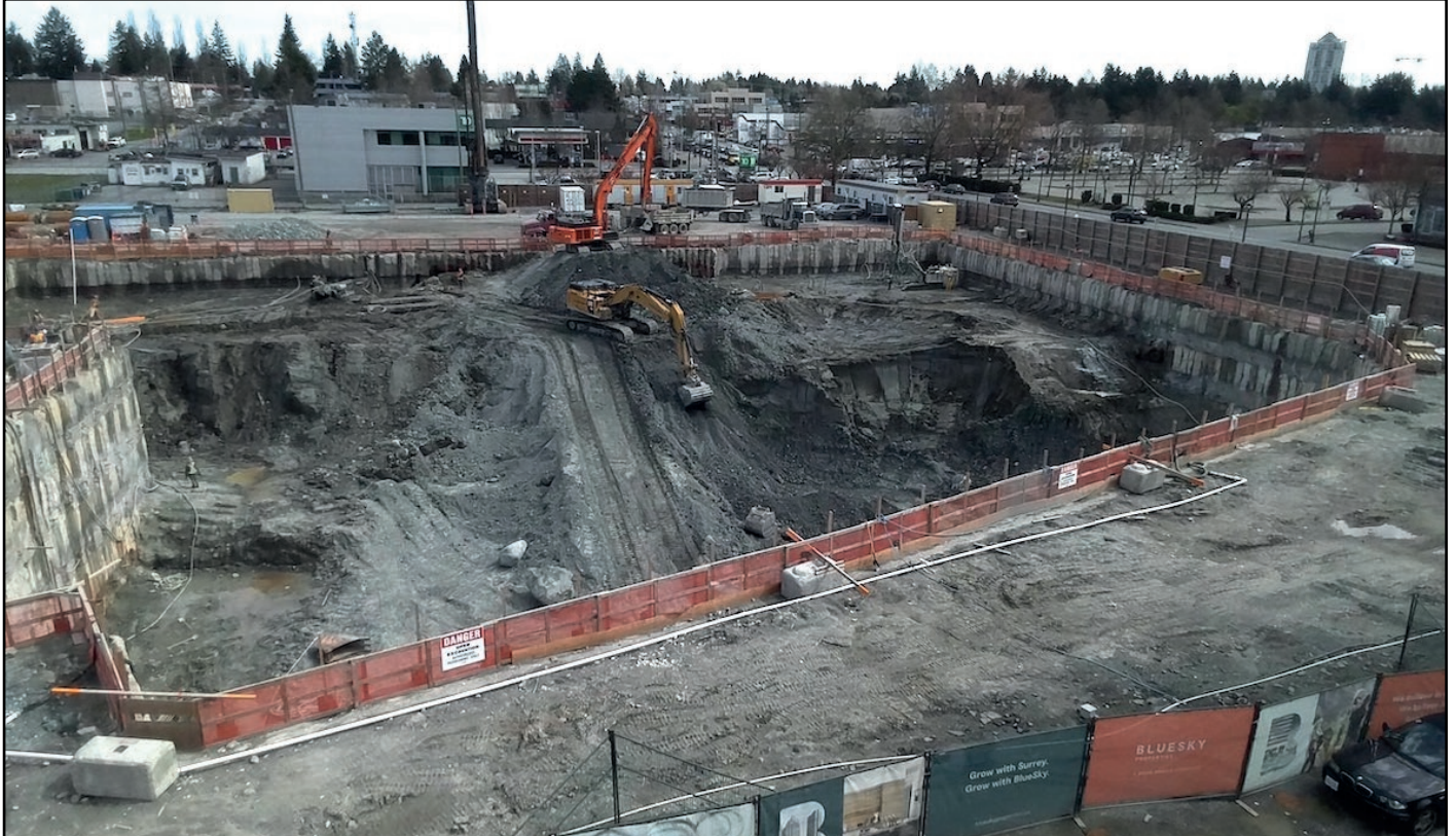
Parkway (Phase 1) - Excavation progressing
