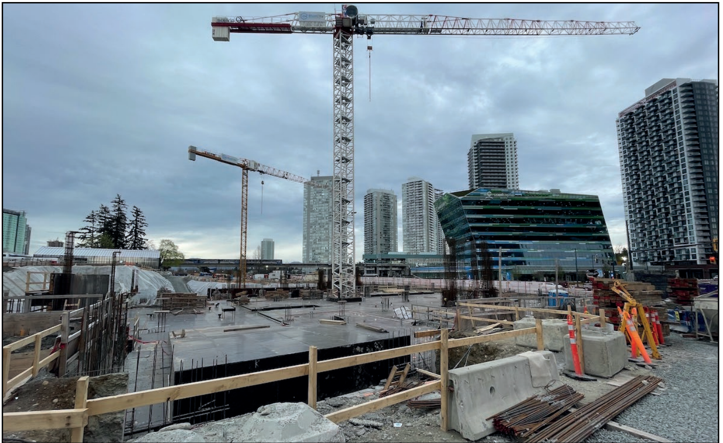
Century City (Phase 1) - Now at grade with work beginning on level 1
