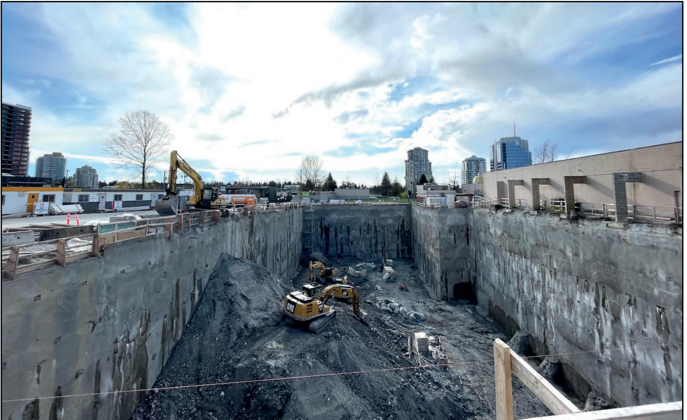
The Grand - Excavation nearing bottom
