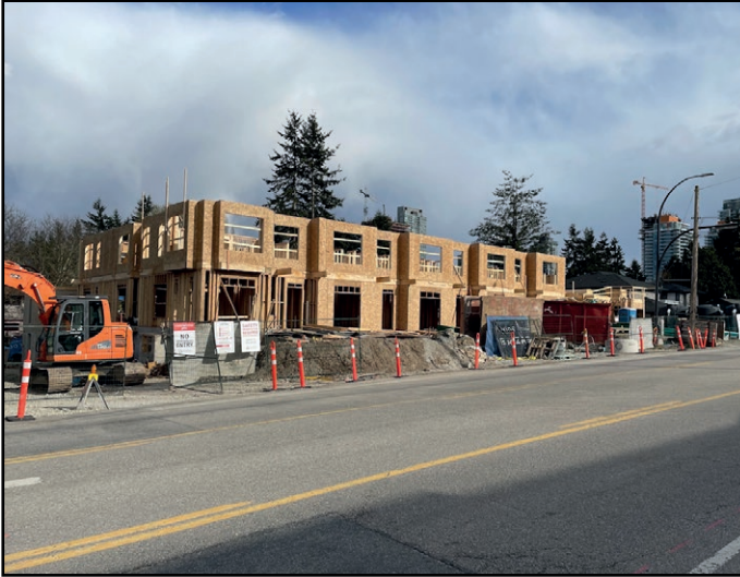
Briza - Now above grade with work progressing on 2nd floor
