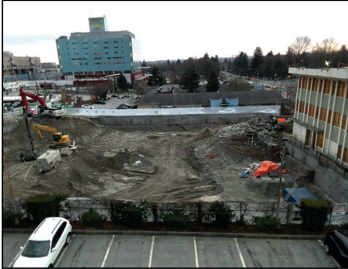
Comma - Excavation progressing
