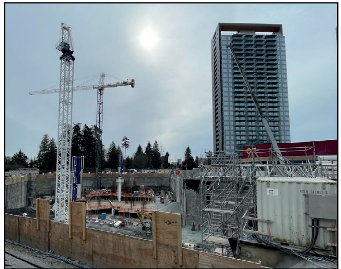
Plaza One & Two - Parking levels construction underway
