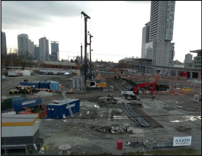
Parkway - Excavation work progresses for tower 1
