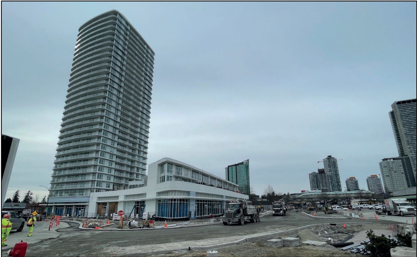
Georgetown One - Road construction underway for new 102A Ave
