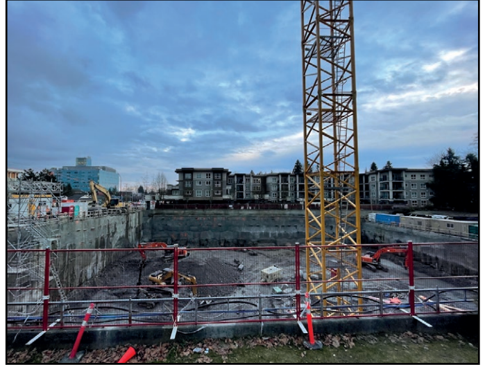
Belvedere - Excavation continues with crane now installed
