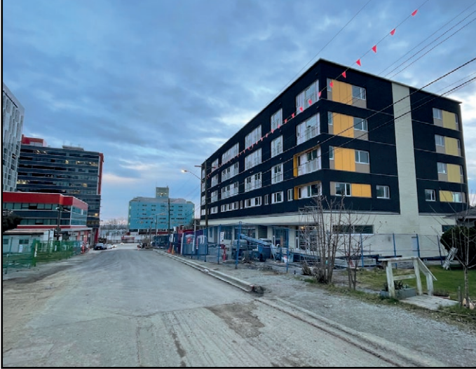
Rosewood - Colour panelling installation now underway
