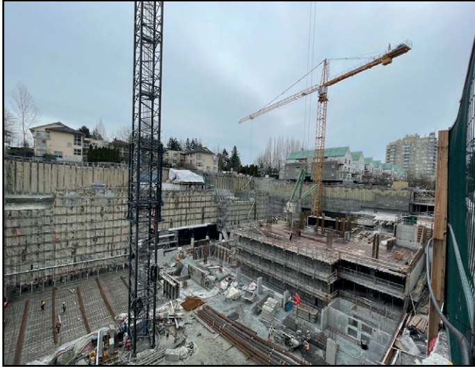
Park George - Parking levels construction nearing grade
