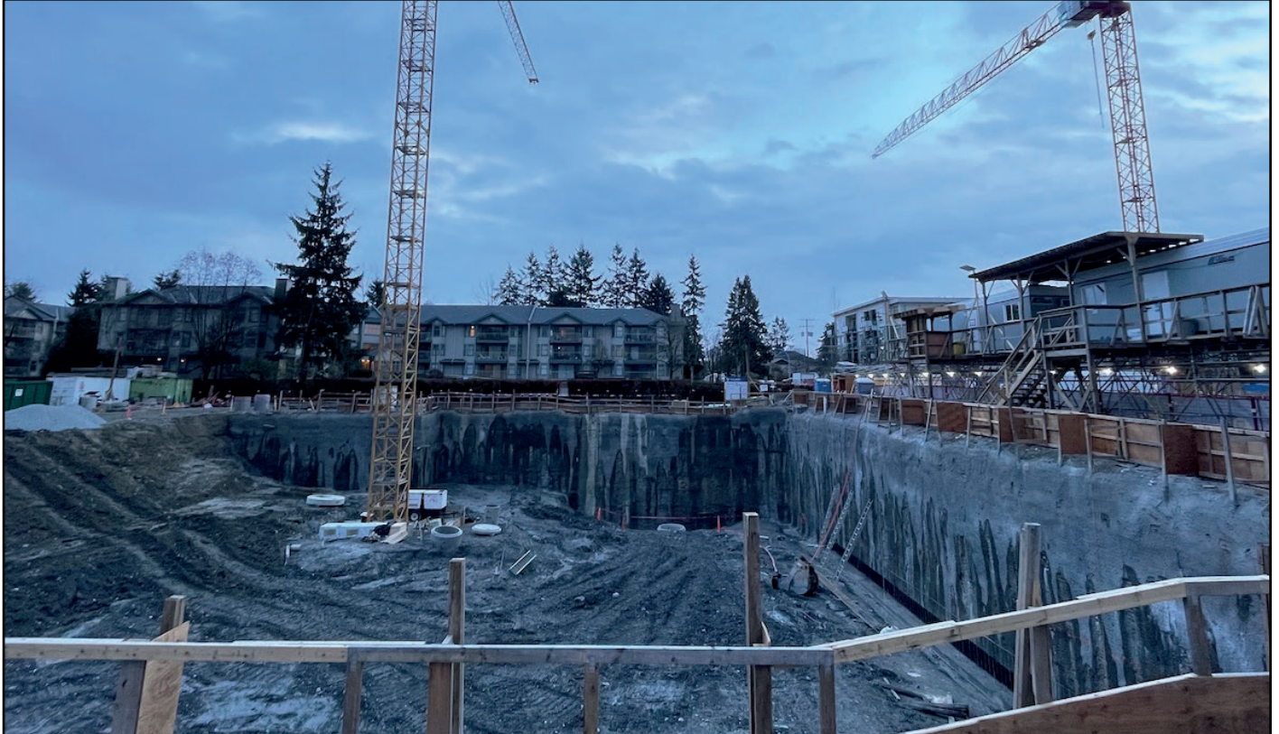
Hendrix - Excavation progressing with crane now installed
