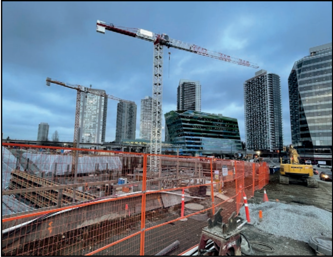
Century City Holland Park - Crane 2 now installed
