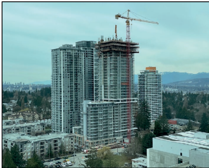
One Central - Continuing to rise with 9-stores remaining
