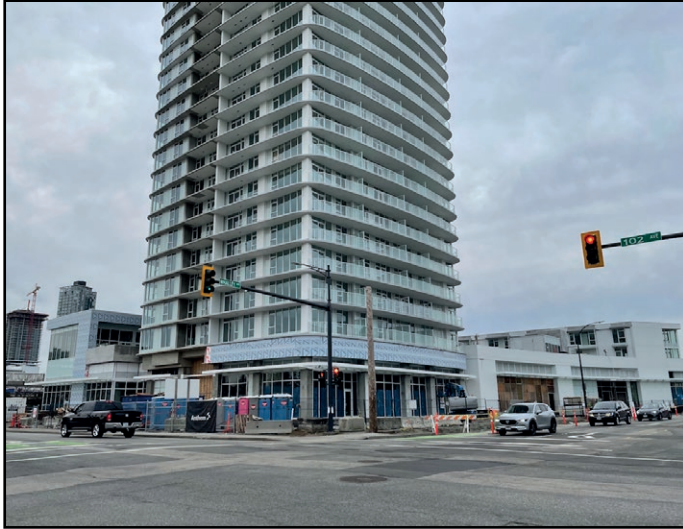
Georgetown One - Corner of Whalley Blvd & 102 Ave
