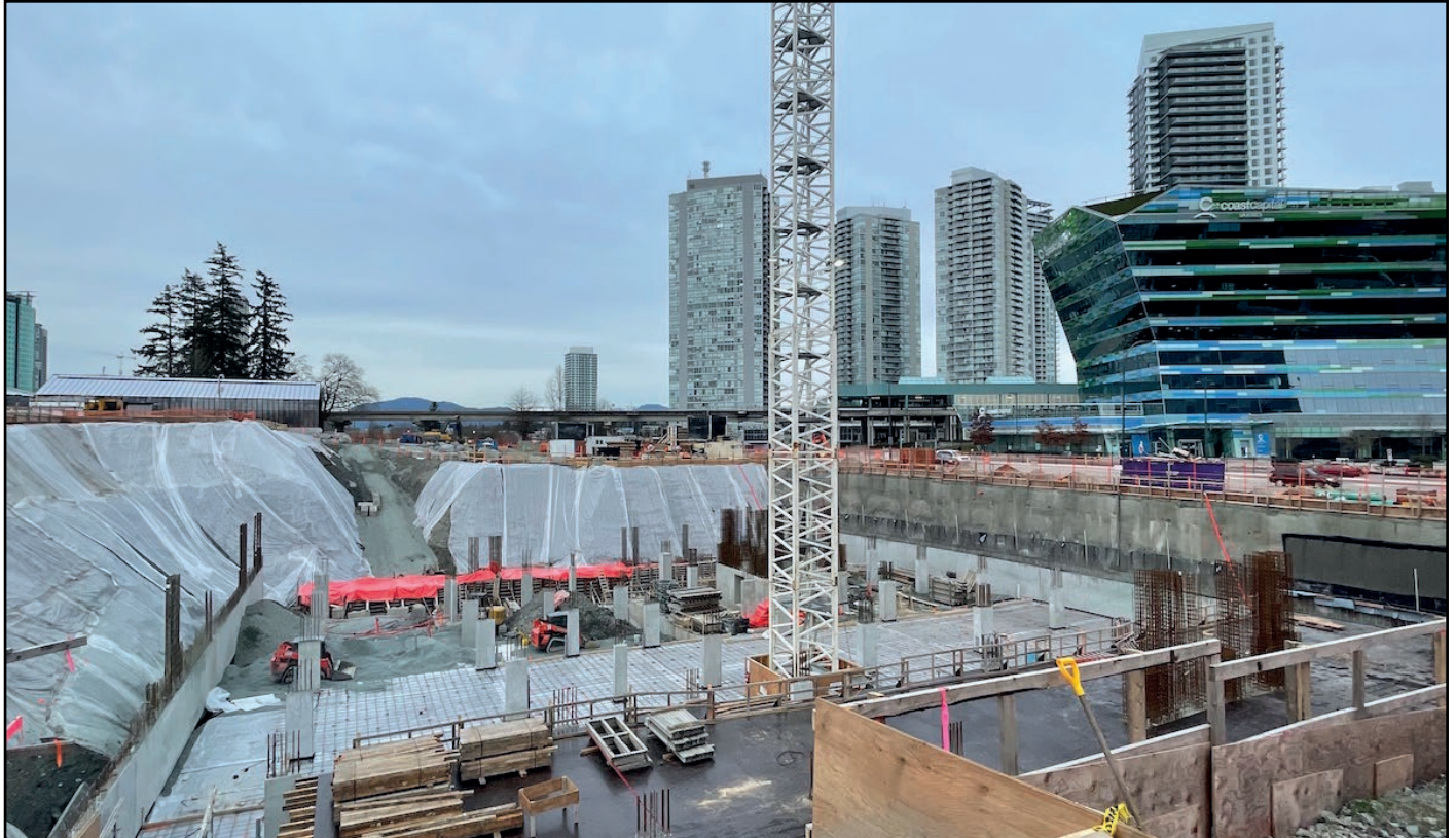
Century City Holland Park - Parking levels construction progressing
