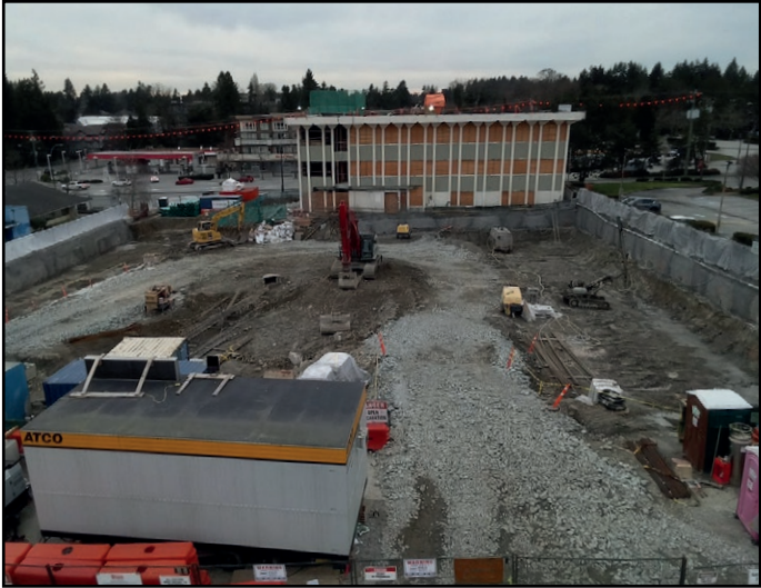
Parks & Yards - Excavation now underway
