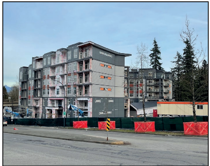
Ledgeview - Exterior work progressing
