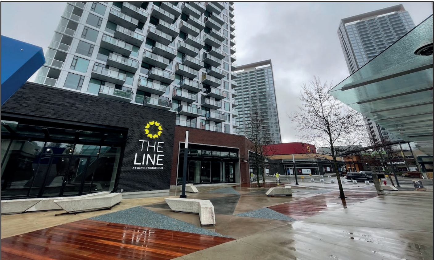
The Line @ King George Hub - 34-storey rental tower with retail has now completed
