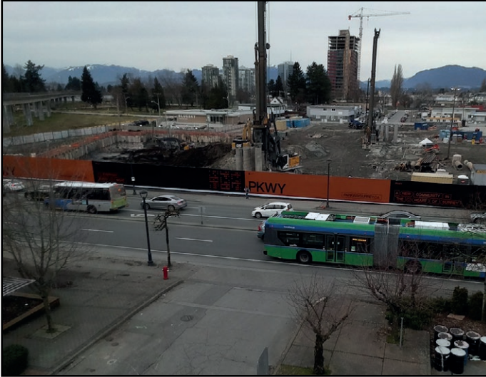
Parkway - Excavation underway for Phase 1 rental tower
