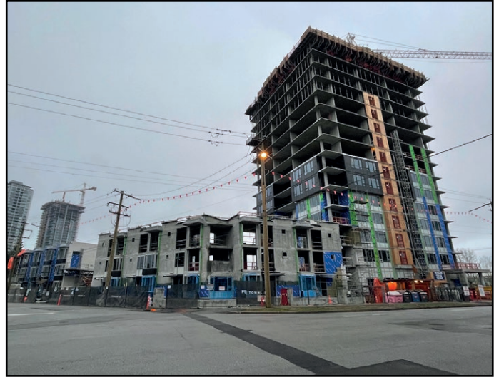
The Holland - Exterior cladding taking shape
