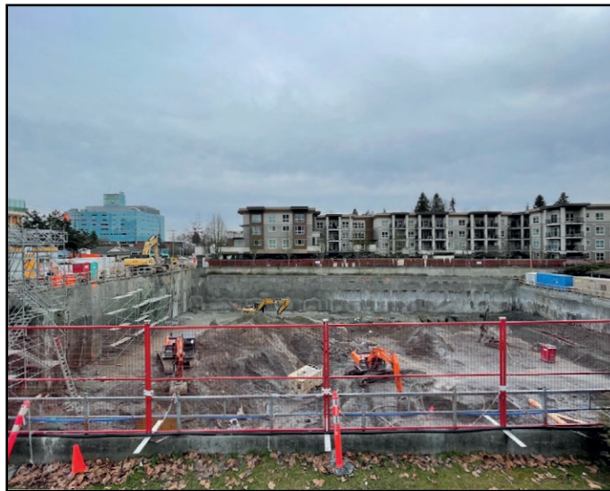
Belvedere - Excavation progressing
