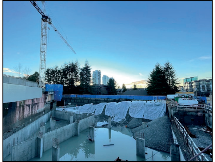
Centra - Underground parking levels taking shape
