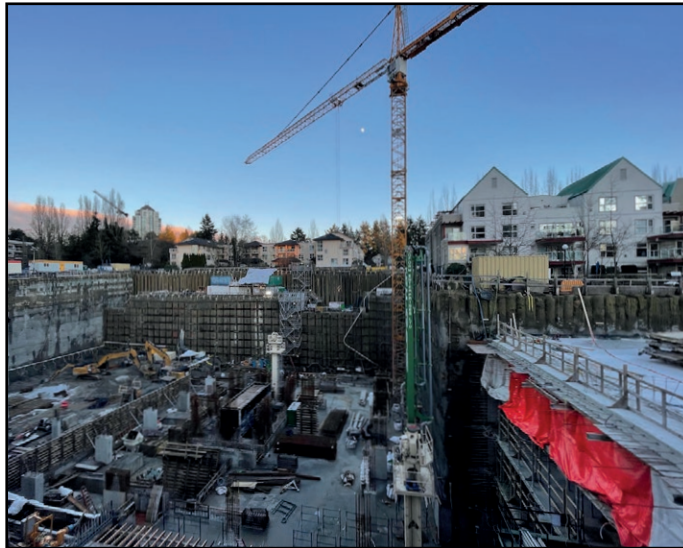
Park George - Underground parking levels progressing
