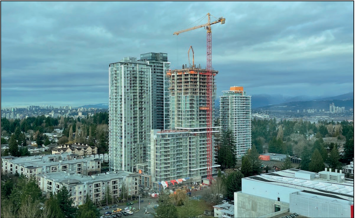
One Central - Continuing to climb to final height of 44-Storeys
