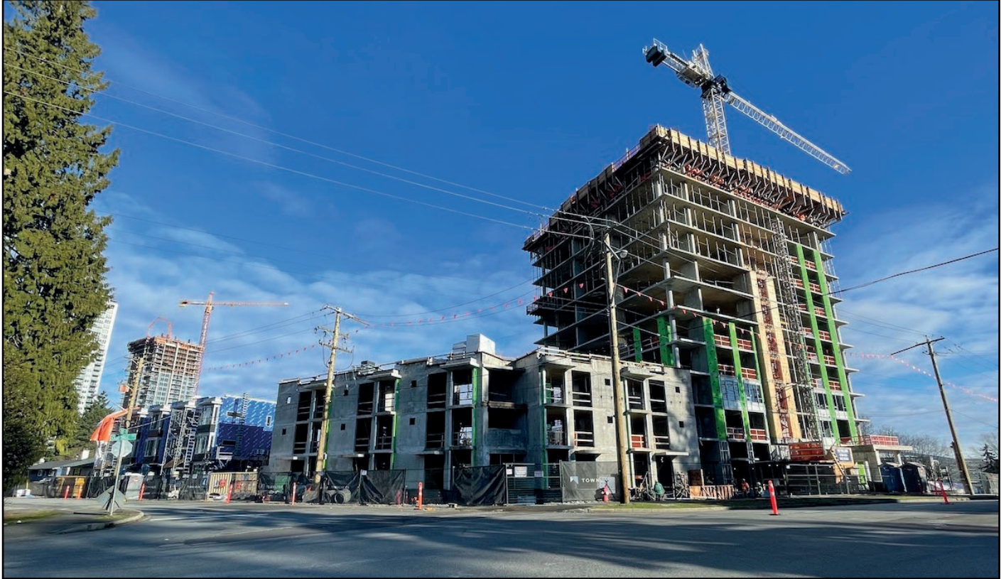
The Holland - Gaining height with glazing installation beginning
