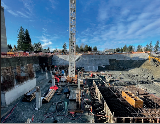
Century City - Underground parking levels taking shape
