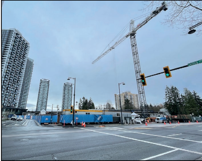
Plaza One & Two - First Crane now installed
