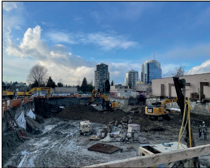
The Grand - Excavation progressing
