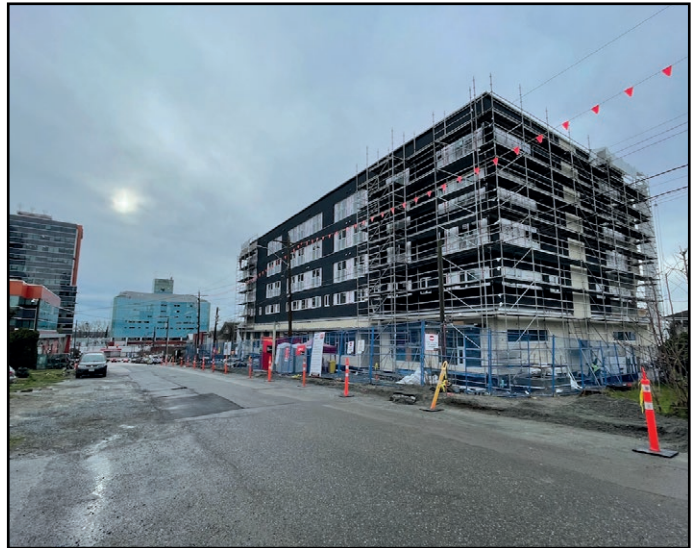
Rosewood - Exterior cladding taking shape
