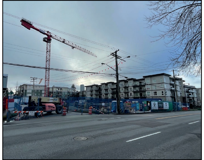
Q5 - Underground parking levels construction underway
