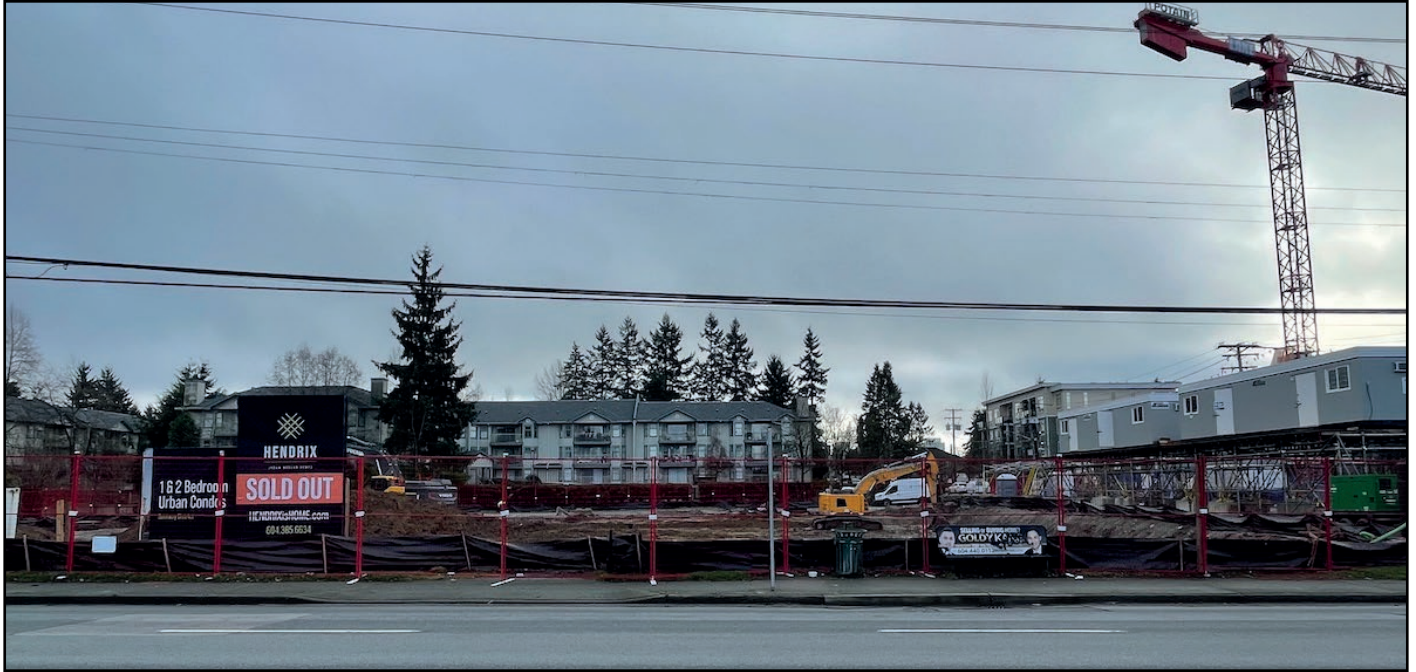
Hendrix (6-Storey Residential) - Excavation now underway on 108 Ave
