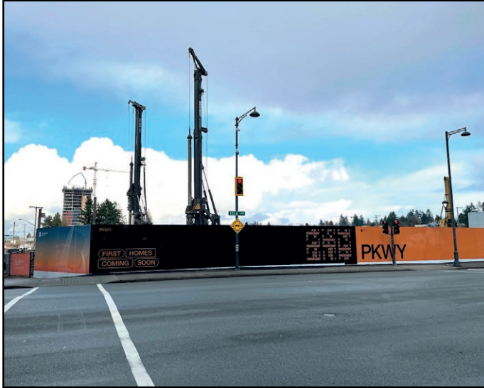
Parkway - Marketing fencing now up along 104 Ave
