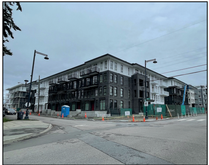
Parker - Nearing completion at 105 Ave & 139 St
