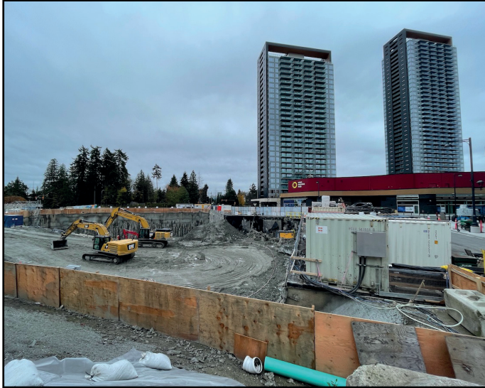
Plaza One & Two - Excavation continues
