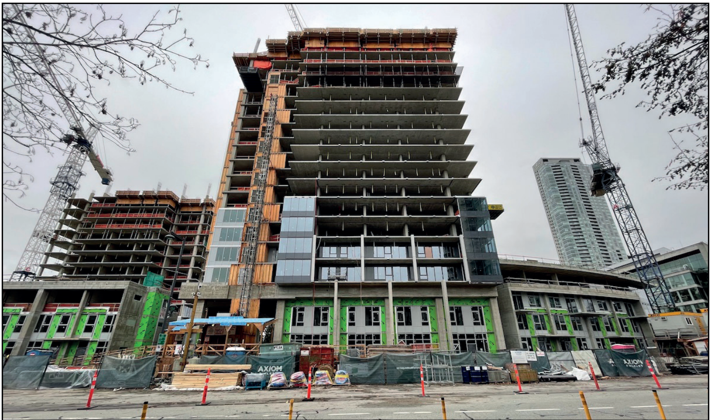
University District - Glazing & cladding taking shape as towers continue to rise
