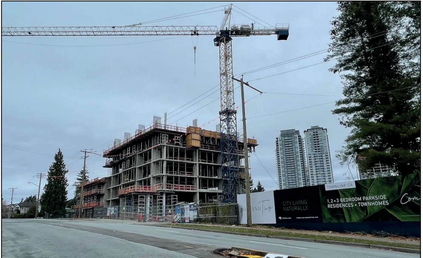
The Holland - Main tower beginning to rise above Old Yale Rd
