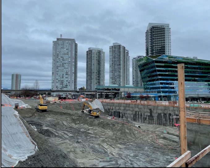
Holland Parkside - Excavation continues
