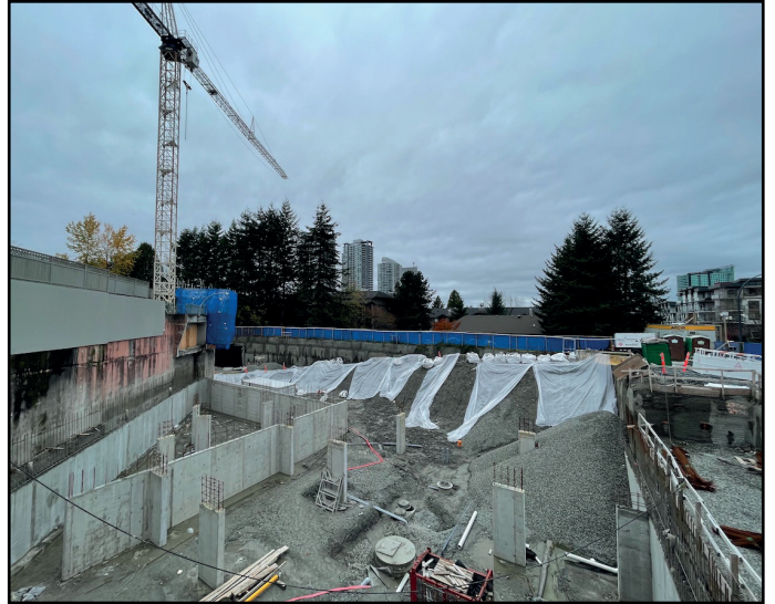
Centra - Foundation and parking level construction underway
