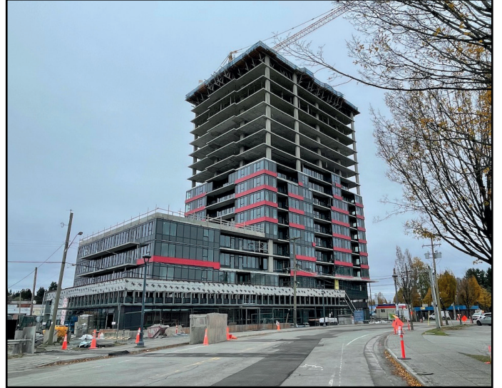
Parc Centrale - Exterior glazing & cladding progressing
