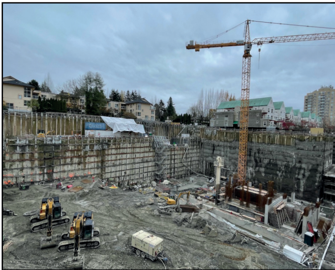
Park George - Excavation and foundational work continues
