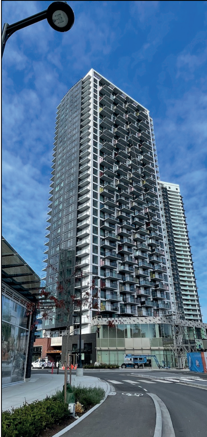
The Line @ King George Hub - Nearing completion
