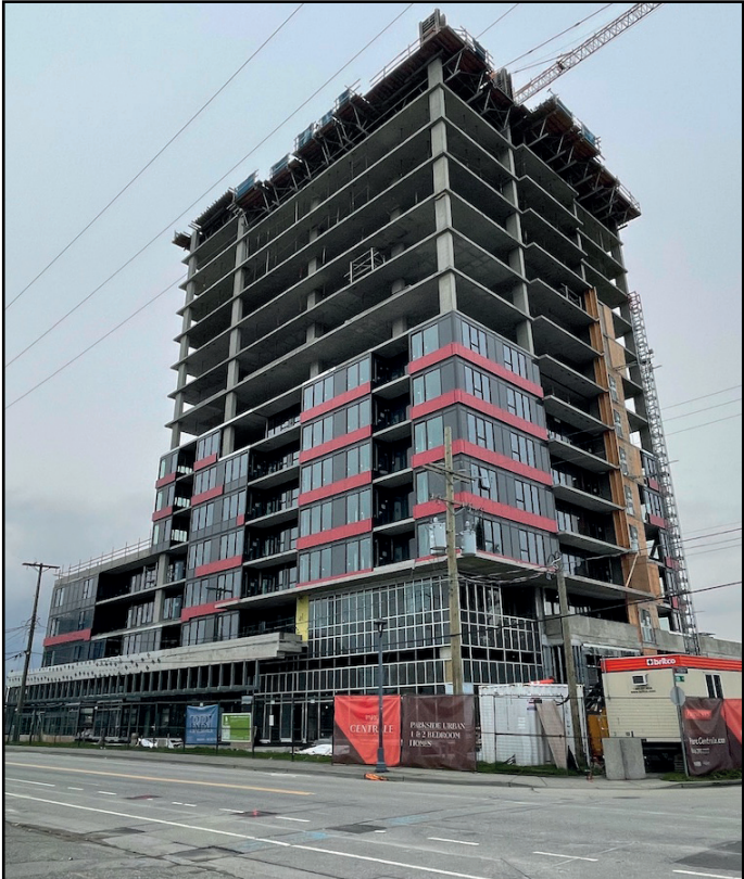
Parc Centrale - Nearing final height with cladding progressing
