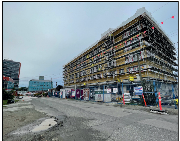
Rosewood - Exterior cladding installation underway
