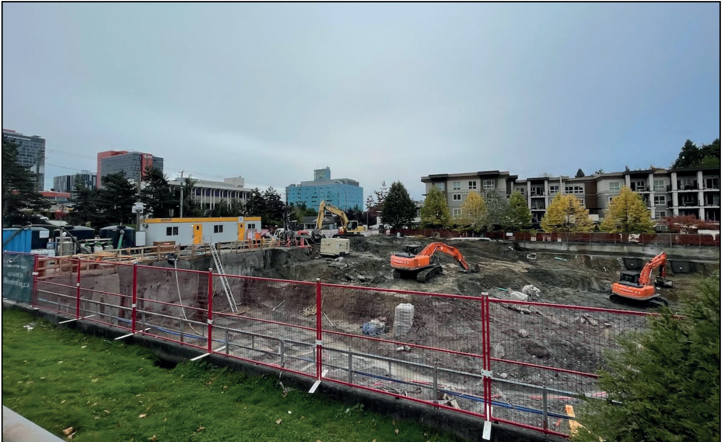
Belvedere - Excavation progressing
