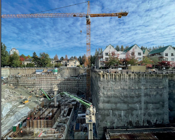
Park George - Foundation and parking levels underway
