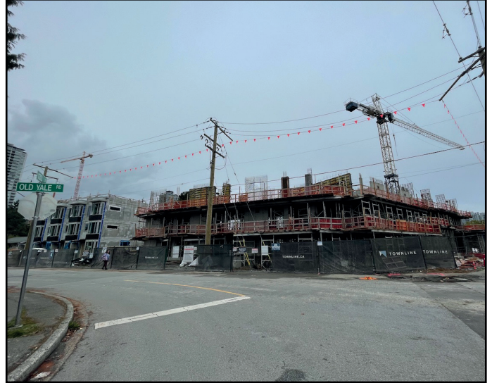
The Holland - Level 3 beginning to take shape
