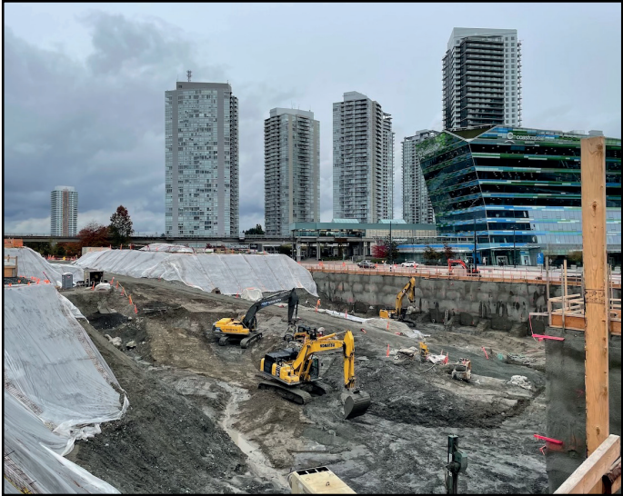
Holland Parkside - Excavation progressing
