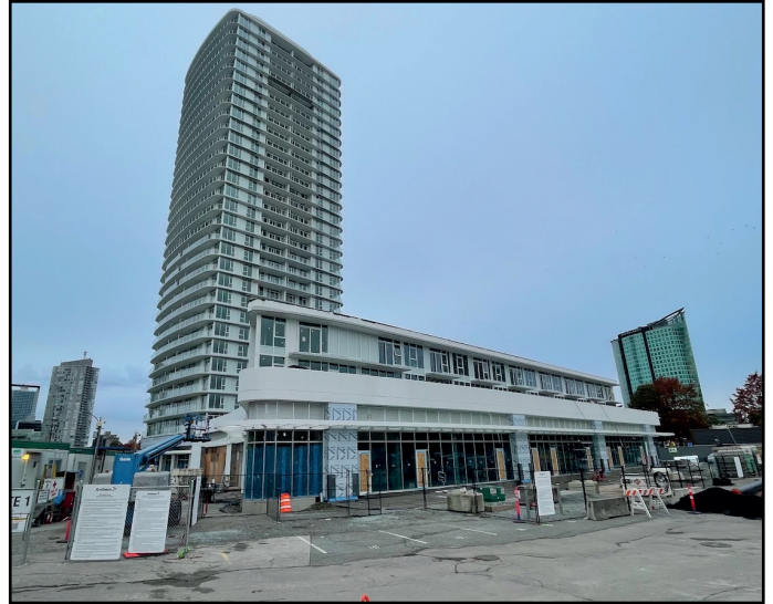
Georgetown One - Work continues on podium and tower
