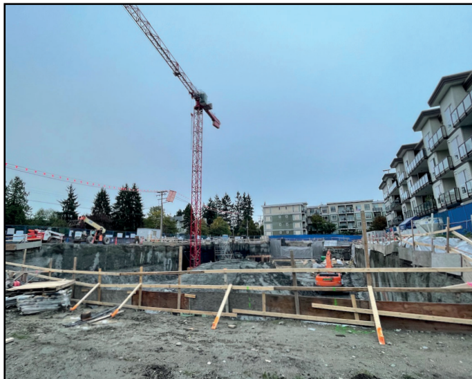
Q5 - Crane now installed
