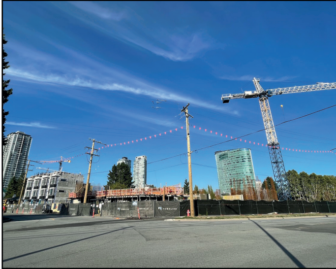
The Holland - Beginning to rise at 133 St & Old Yale Rd
