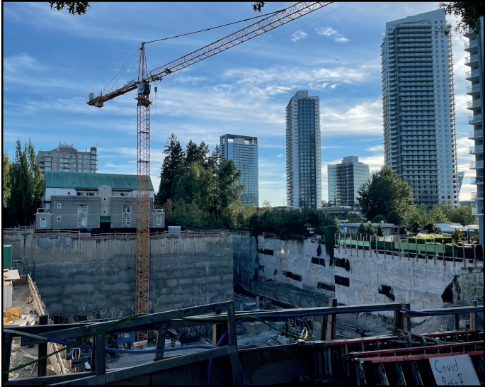
Park George - 1st Crane now installed
