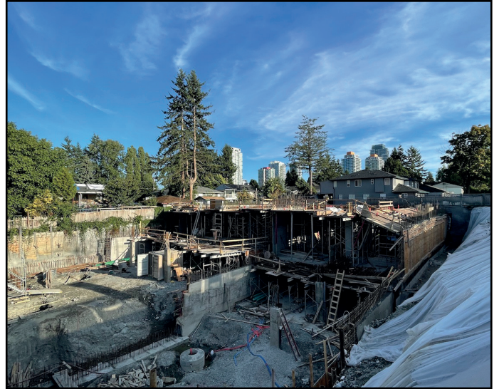
Briza - Work continuing on underground parking levels
