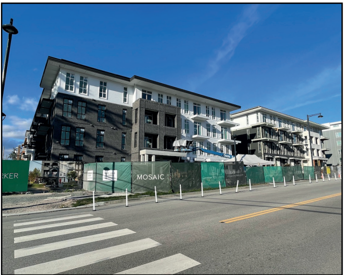
Parker - Exterior cladding mostly complete
