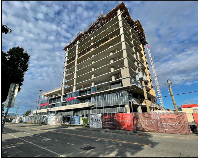
Parc Centrale - Glazing installation underway on lower levels
