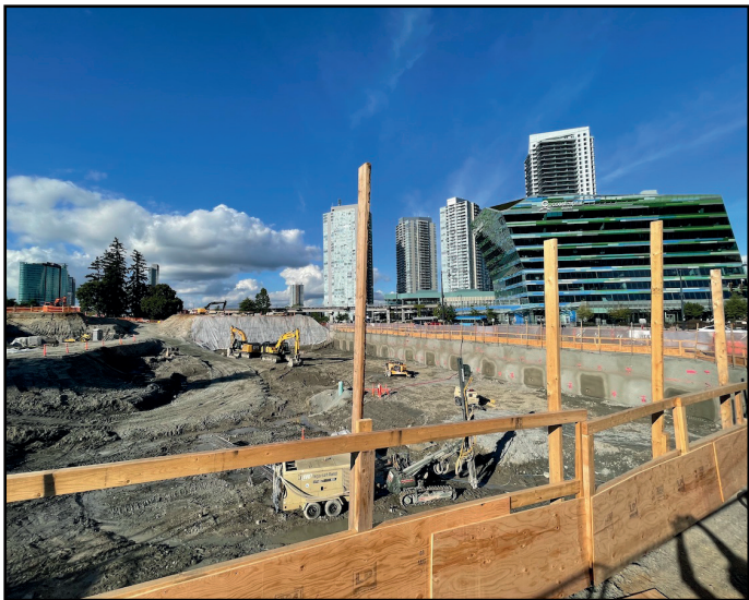
Holland Parkside - Excavation work continues
