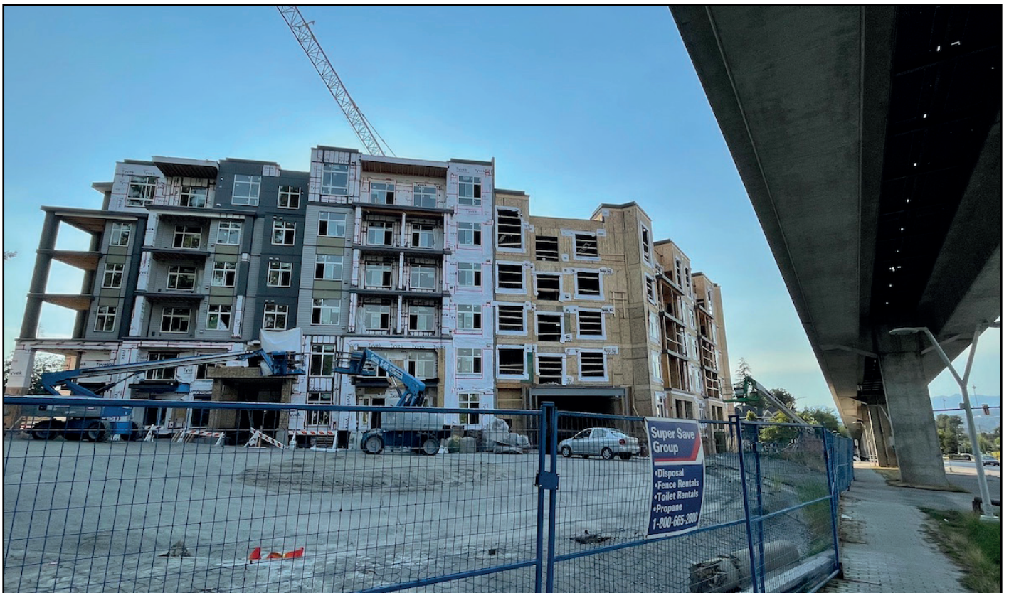
Ledgeview - Topped out at 6-storays with glazing and cladding installation underway
