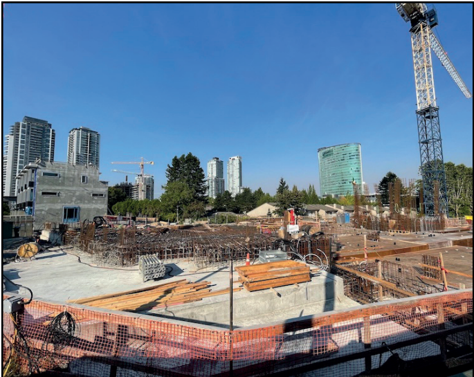
The Holland - Work beginning on level 1 above grade
