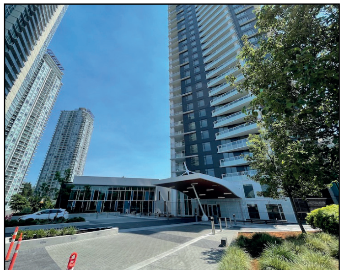
Park Boulevard - Main entry nearing completion
