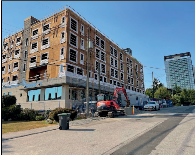
Rosewood - Glazing installation underway
