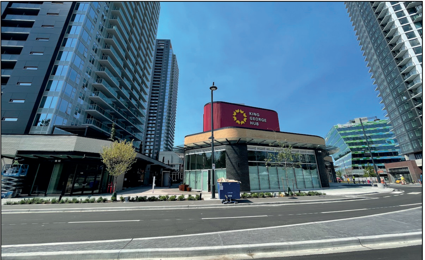
King George Hub - Phase B now substantially complete with residential towers ready for occupancy. Retail and office to follow.
