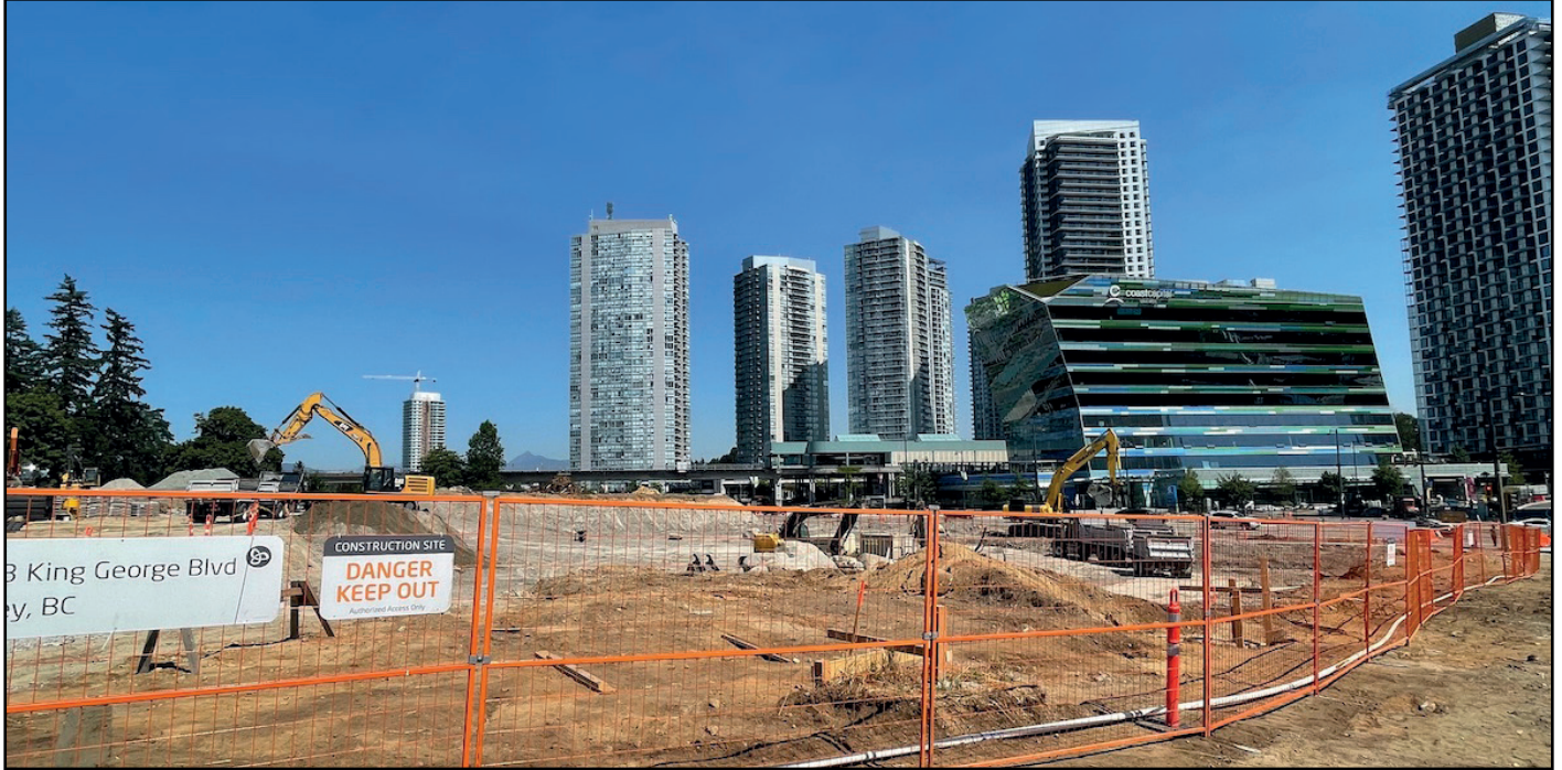
Holland Parkside - Excavation now underway for Phase 1 of Holland Parkside
