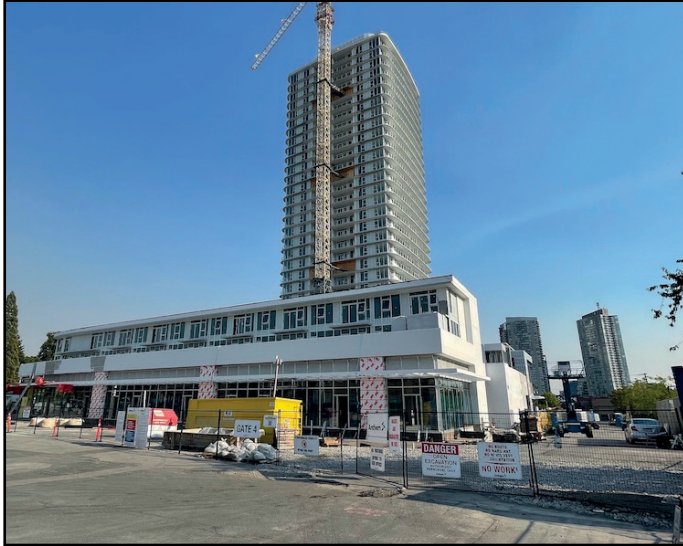
Georgetown One - Construction starting on new 102 Ave
