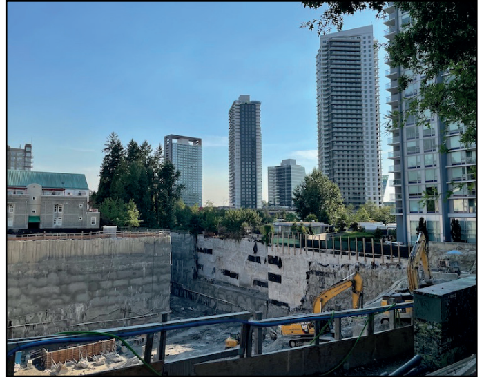
Park George - Excavation pit nearing bottom
