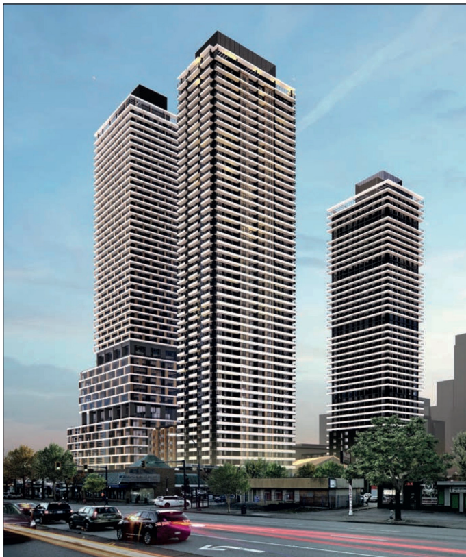
View looking south-west from King George Blvd towards Tower 3
