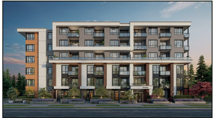
Hendrix - 6-Storey (86 Unit) condominium project by Sync Properties located at 108 Ave & 138 St
