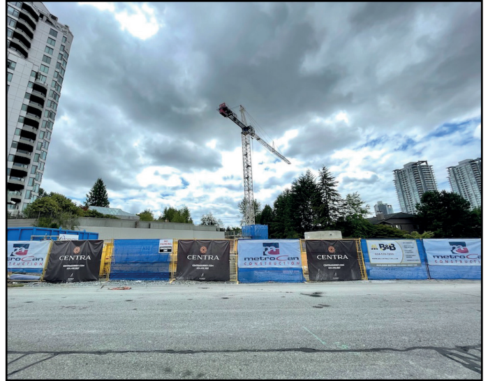
Centra - Crane now installed
