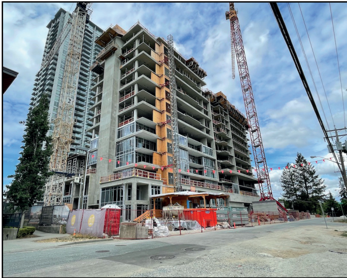
One Central - Glazing installation now underway on podium
