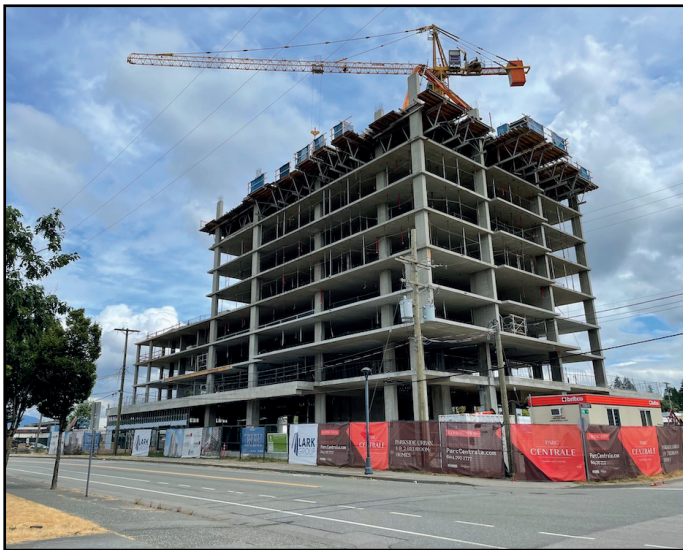
Parc Centrale - Continuing to rise at City Parkway & 106 Ave
