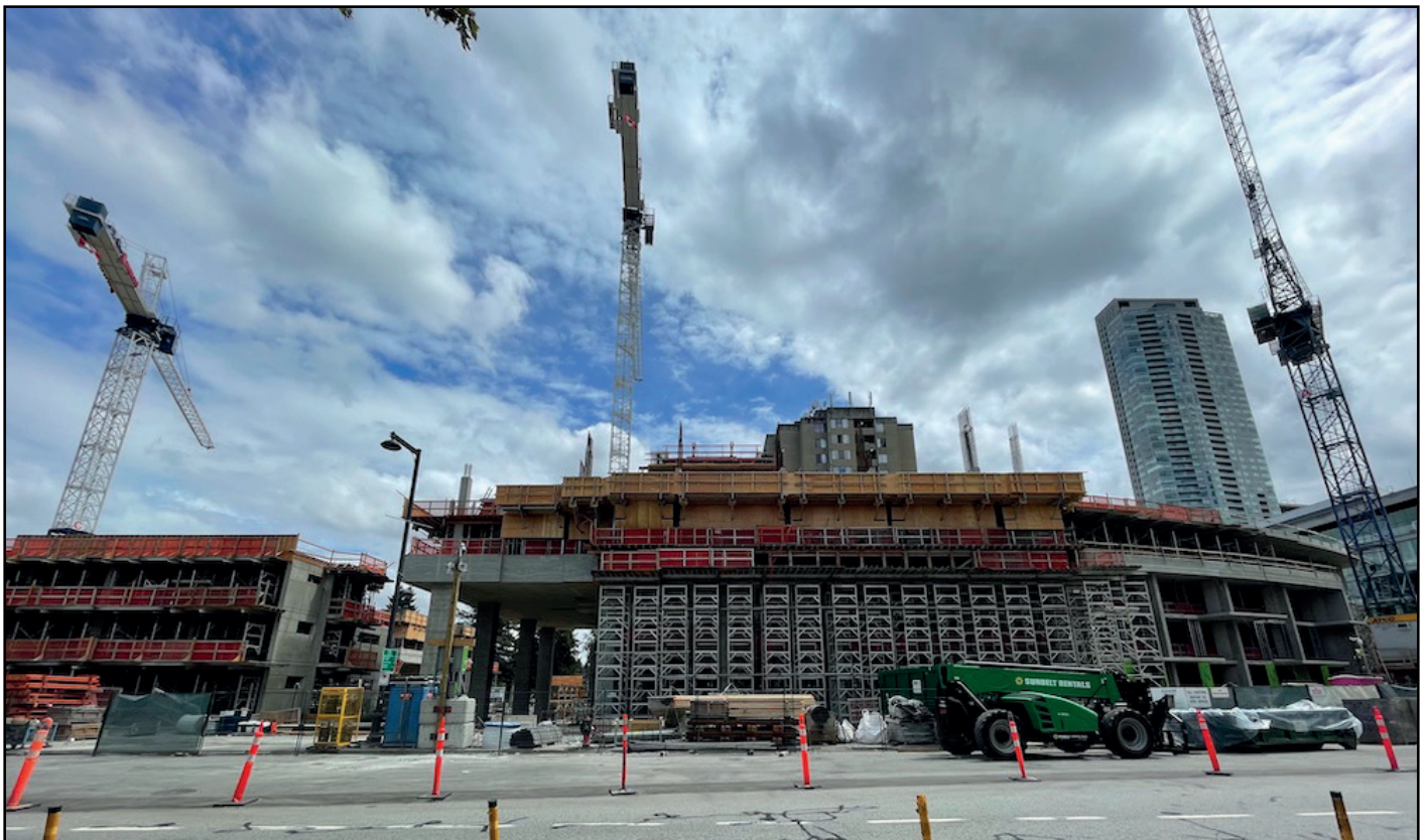
University District - Construction of podium levels underway along University Dr
