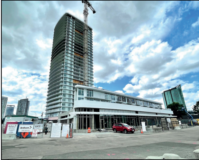
Georgetown One - Work continues on main tower and podium
