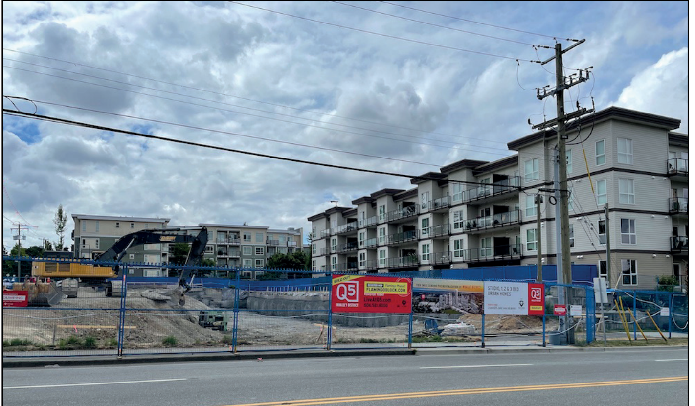
Q5 - Excavation now underway
