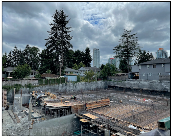
Briza - Parking levels construction nearing grade
