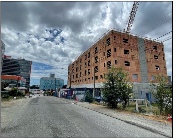
Rosewood - Building frame now topped off at level 5
