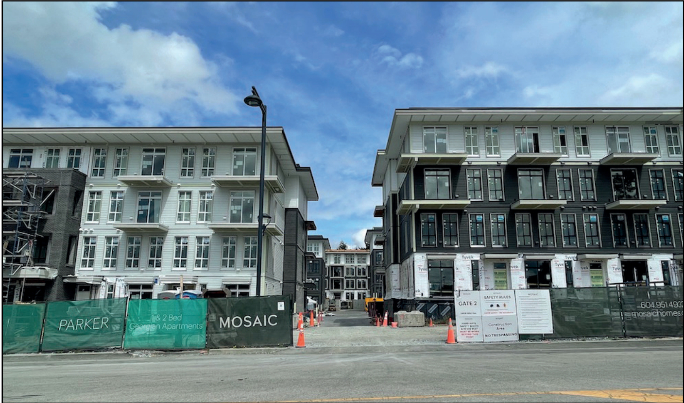
Parker - Exterior work continues View along 105 Blvd
