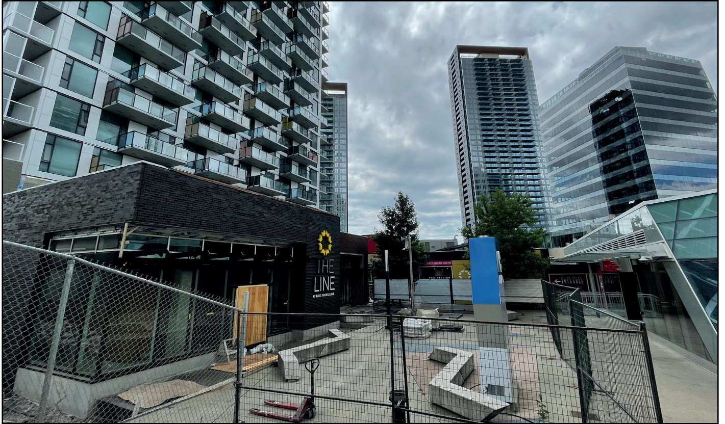
King George Hub - Rental tower 'The Line' nearing completion
