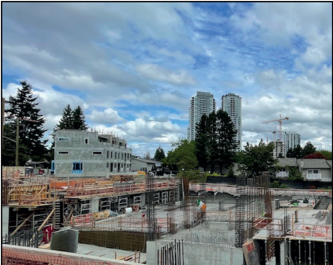
The Holland - Parking levels construction nearing grade
