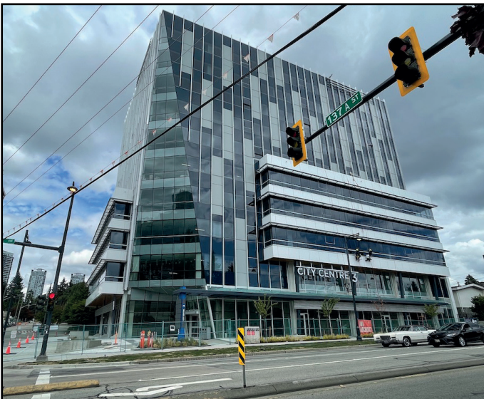
City Centre 3 - 10-Storey Office & Retail now complete
