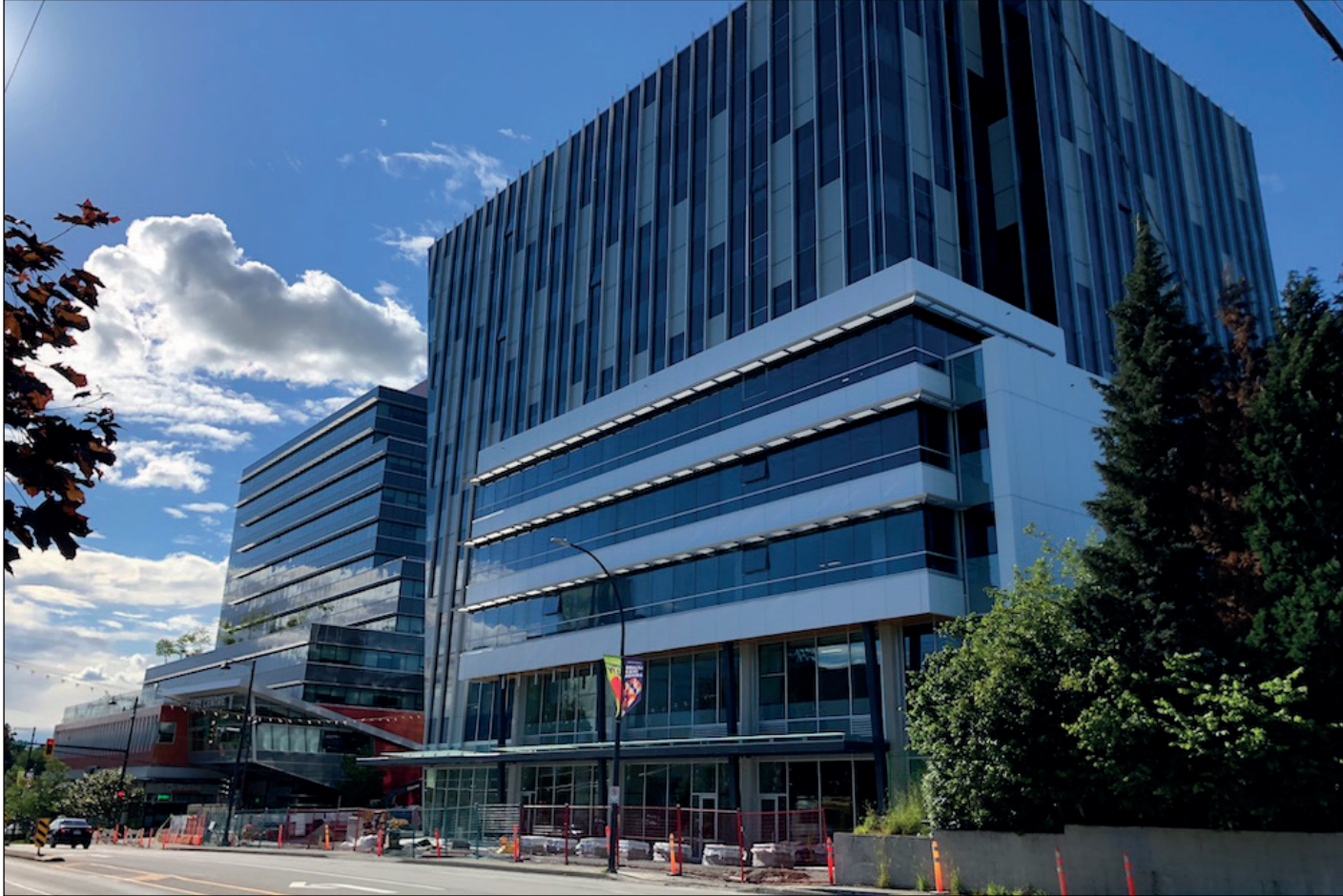
City Centre 3 nearing completion on 96 Ave across from Surrey Memorial Hospital
