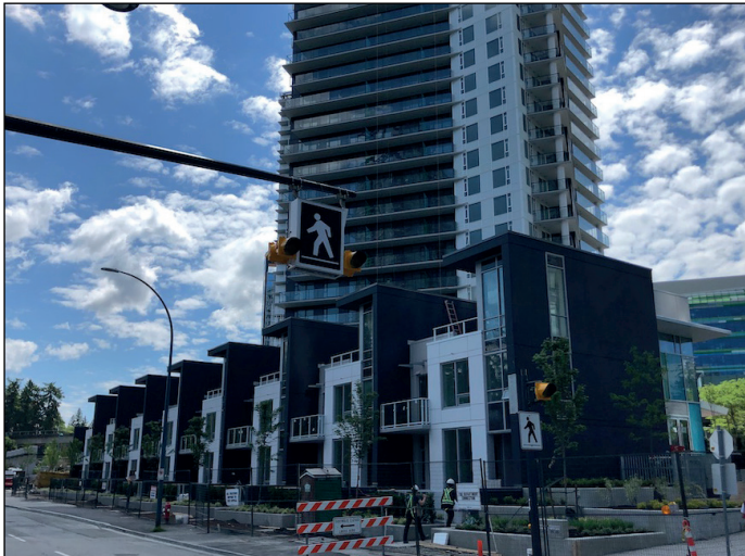
Park Boulevard nearing completion on Whalley Blvd near 100 Ave
