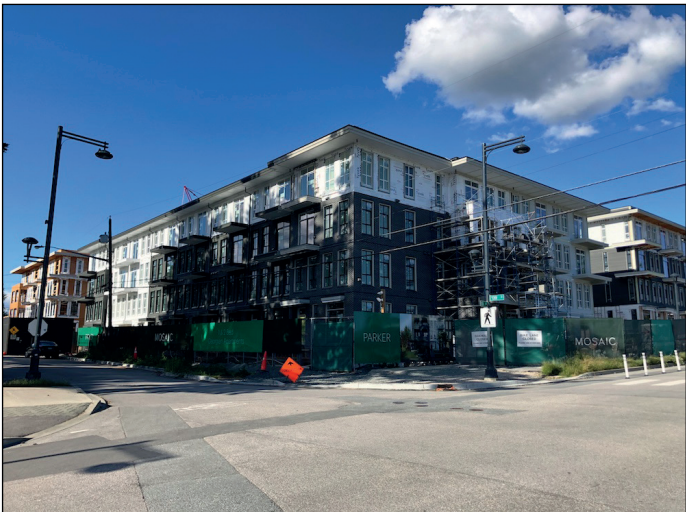
Exterior progress on Parker at 105 Ave & 139 St
