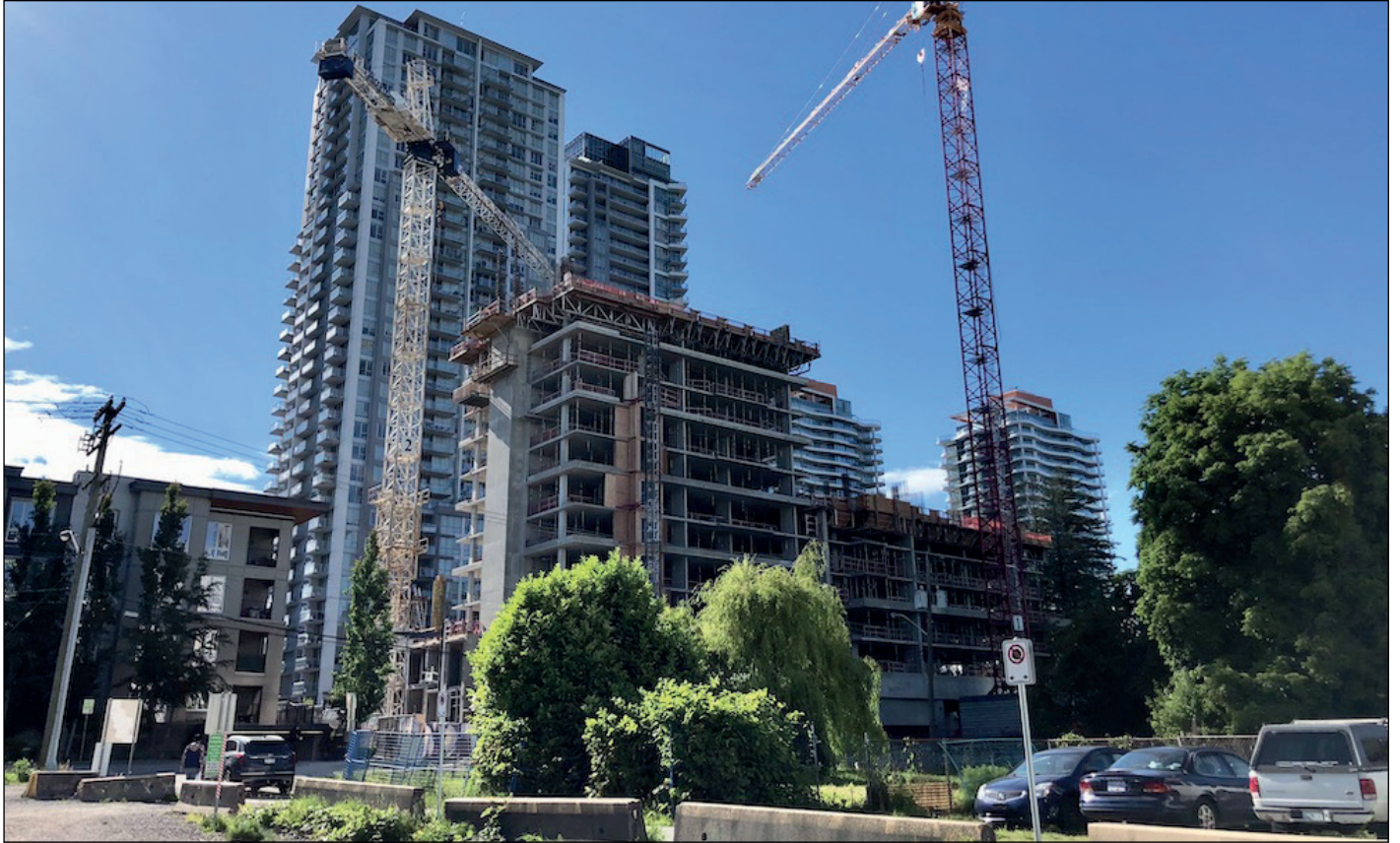
One Central rising in West Village
