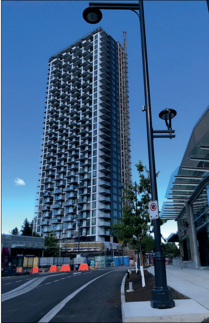
King George Hub (Phase C) Rental Tower nearing completion
