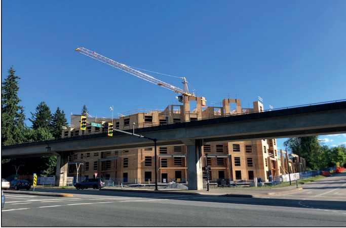
Ledgeview (formerly La Voda) rising at 132 St & King George Blvd
