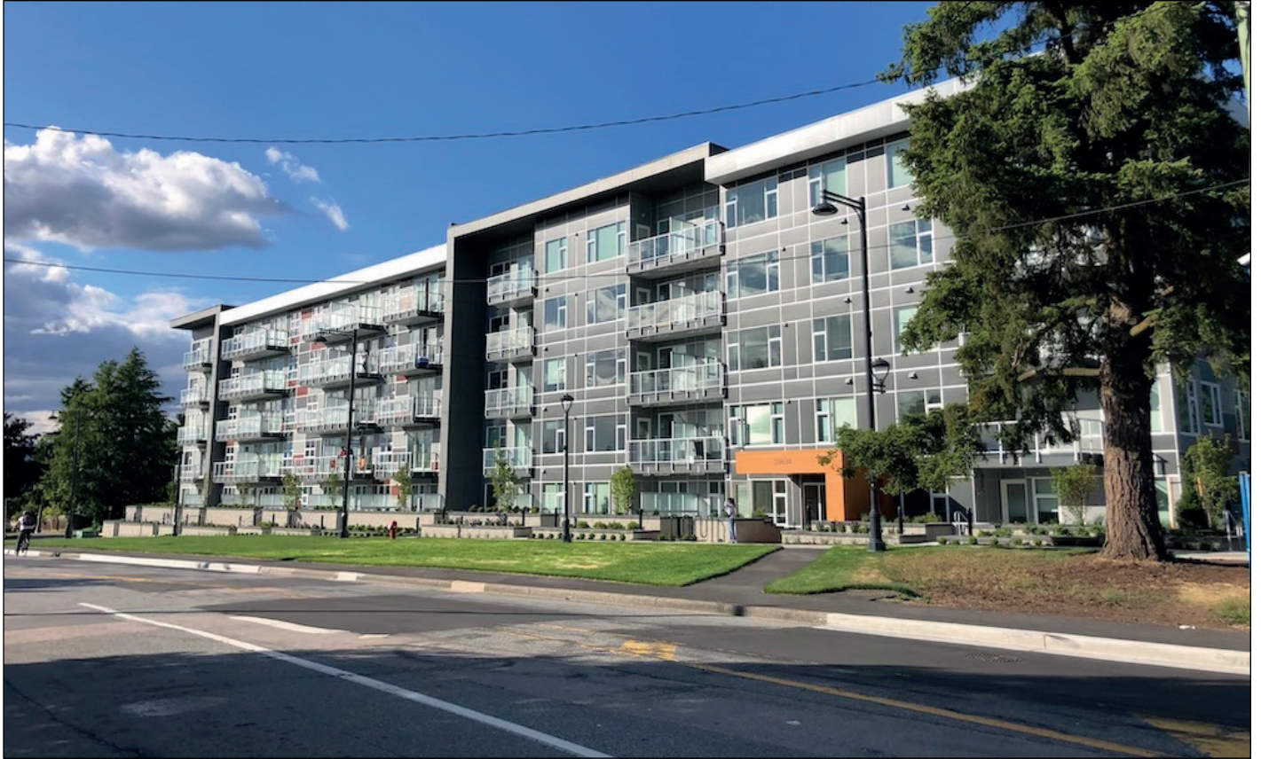
Maverick at Whalley Blvd & Grosvenor Rd completed in May
