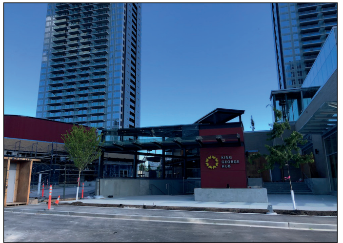
King George Hub retail plaza nearing completion
