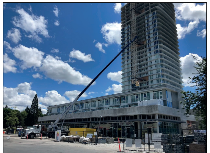
Glazing installation underway on Georgetown retail / townhouse podium
