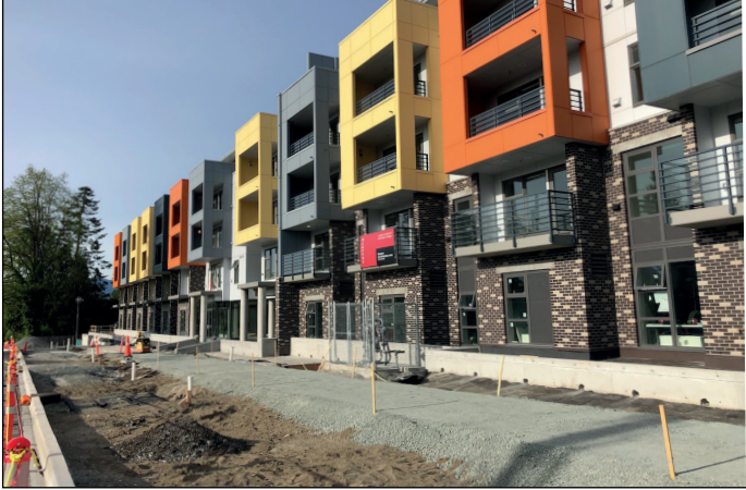
Street frontage upgrades underway along 132 St at Camellia Seniors Living
