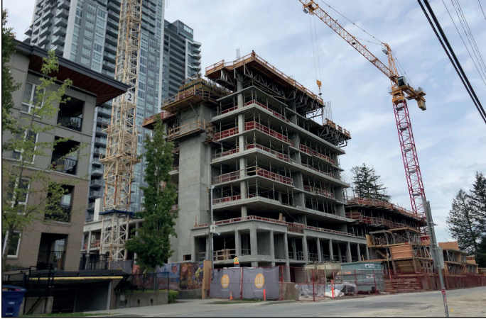
North-west view of One Central's podium along 133A St
