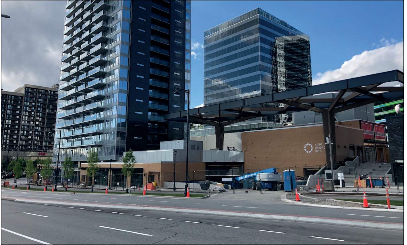
King George Hub nearing completion along Fraser Highway
