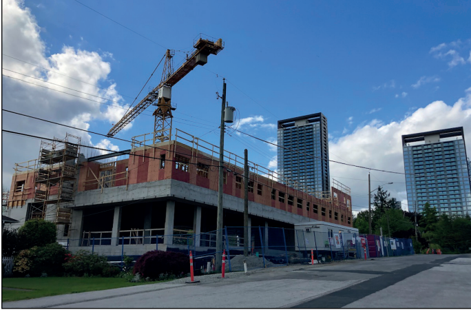
Rosewood Transitional Housing Project rising on 137 St
