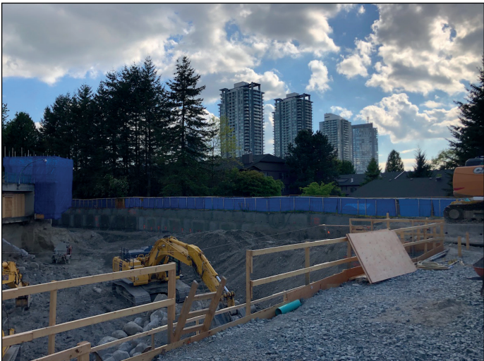
Excavation underway for Centra on 101 Ave
