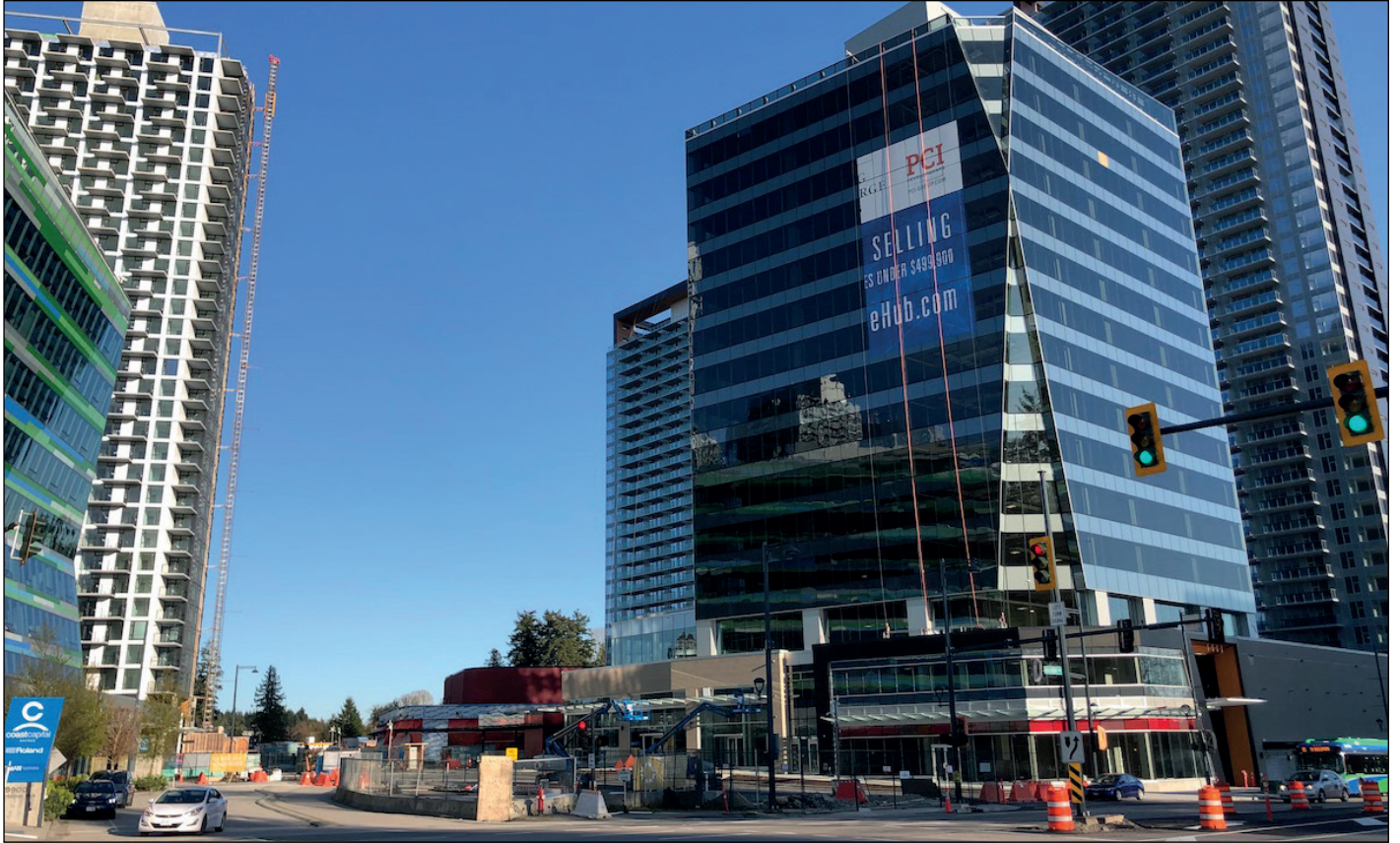
King George Hub office tower nearing completion at new intersection of King George Blvd and George Junction
