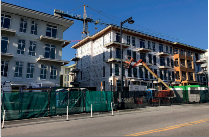
Parker by Mosaic progressing on 105 Ave near 140 St
