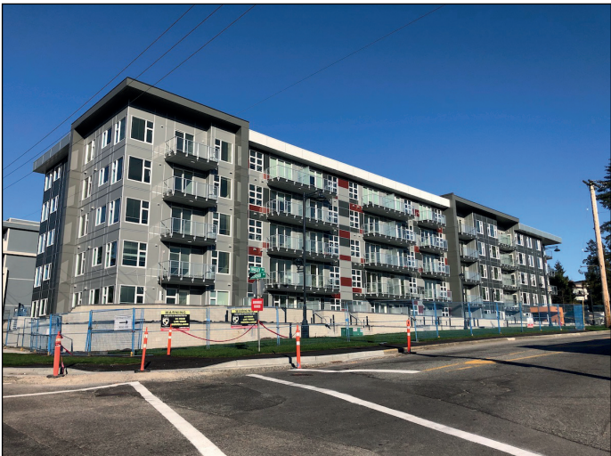
Maverick nearing occupancy at Whalley Blvd & Grosevnor Rd
