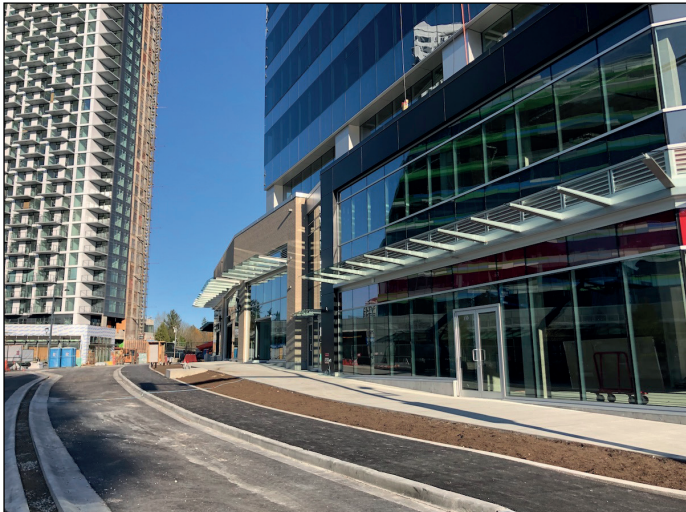
New road, bike path, and sidewalk along George Junction
