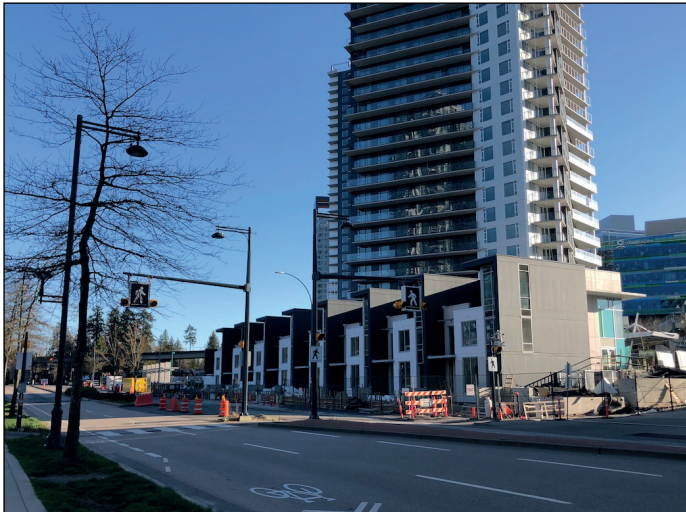
41-Storey Park Boulevard nearing completion along Whalley Blvd
