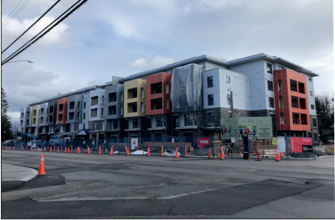
Colourful cladding installation at Camellia Seniors Living - 132 St & 109 Ave
