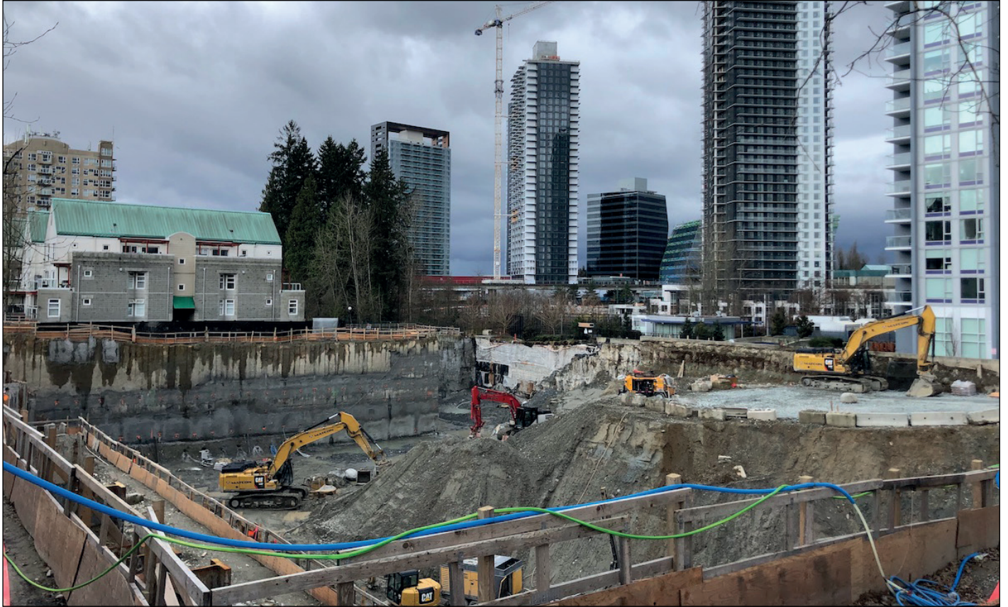
Excavation underway at Park George on 100 Ave
