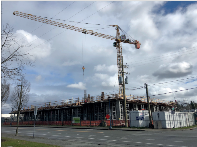
Legion Veterans Village rising above ground at City Parkway & 106 Ave
