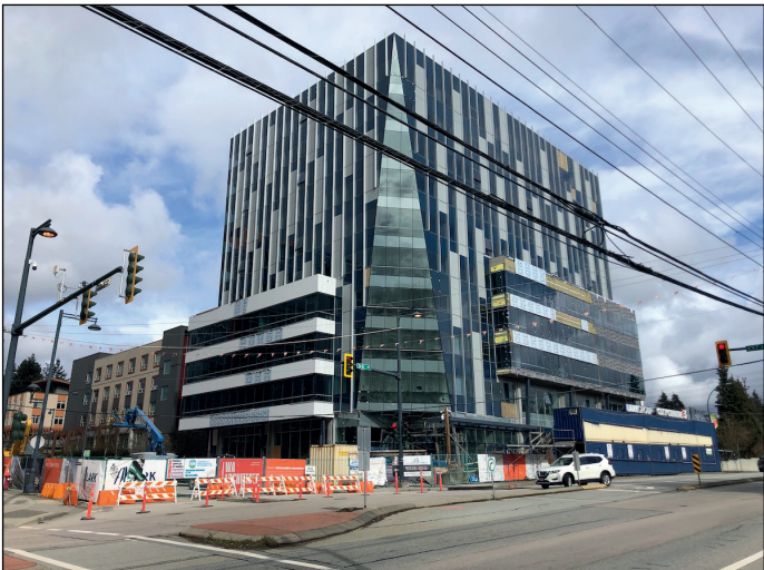
City Centre 3 nearing completion at 96 Ave & 137A St
