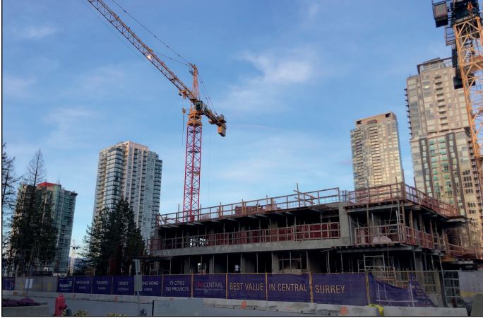
Surrey's next tallest - One Central beginning to rise in West Village
