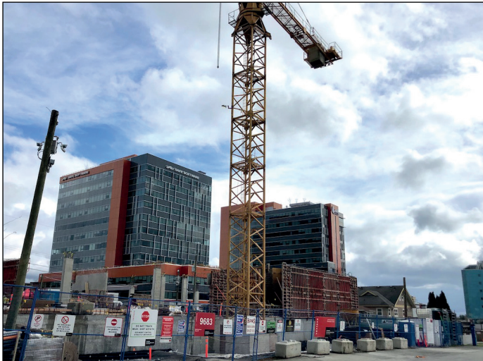
Rosewood Supportive Housing project rising above ground on 137 St
