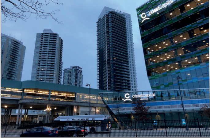
Park Boulevard | 41-Storey Residential | Whalley Blvd & 100 Ave
