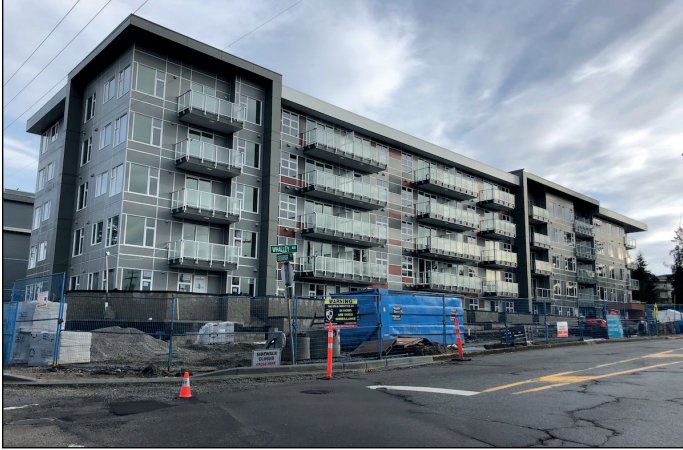
Maverick | 5-Storey Residential | Whalley Blvd & Grosvenor Rd
