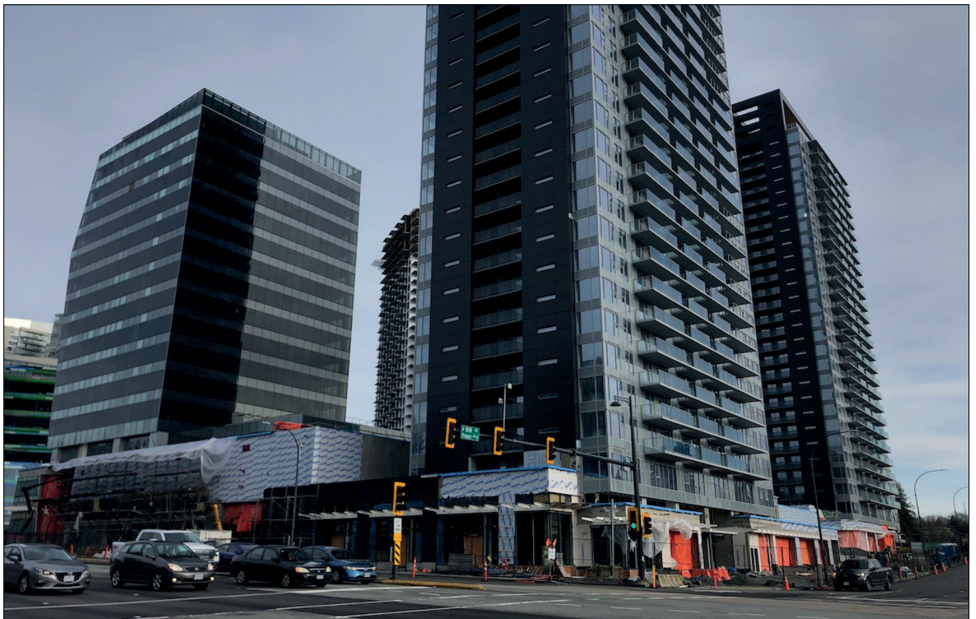
King George Hub Phases B & C | 29 + 34 + 40-Storey Residential, 15-Storey Office, Retail | King George Blvd & Fraser Hwy
