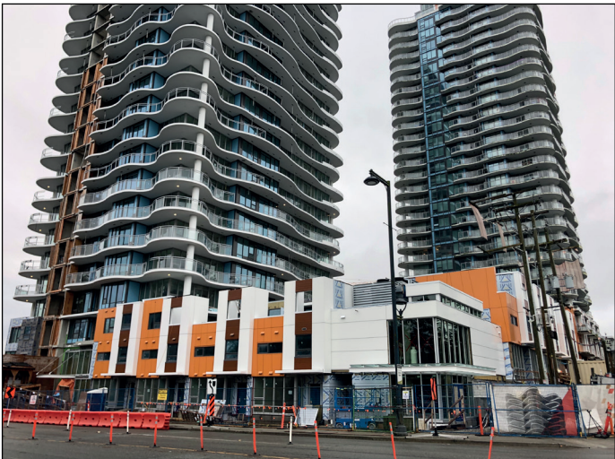
Linea | 28-Storey Residential | 133 St & 104 Ave
