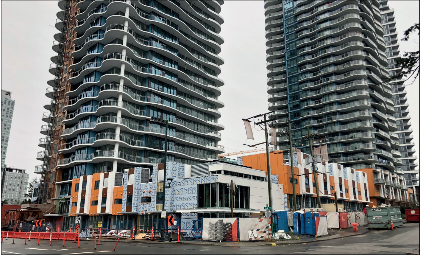
Linea - 28-Storey Residential
