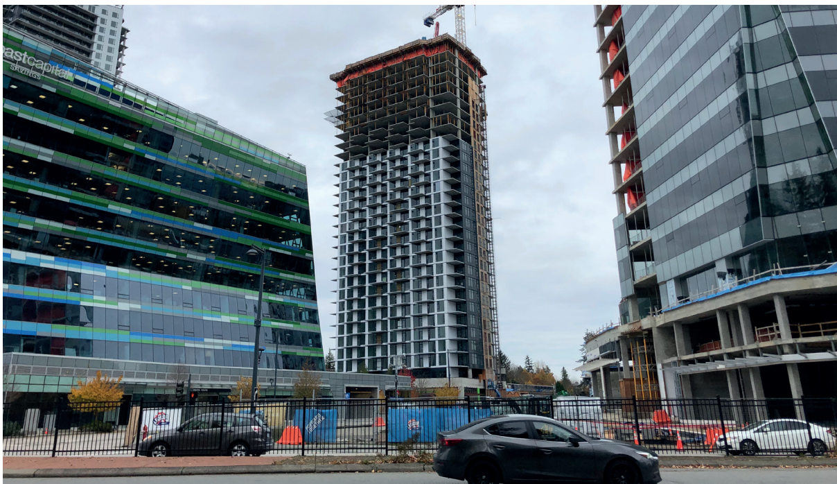
King George Hub (Phase C) - 34-Storey Rental Residential, Retail
